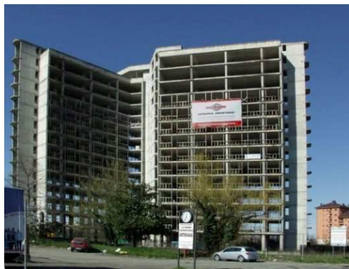
111. Scheletro in cemento del "Blue Residence"
