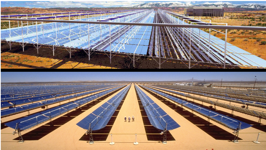
Figure 4.11 – Differences in land coverage density between linear Fresnel reflectors (upper portion) and parabolic trough concentrators (lower portion)
