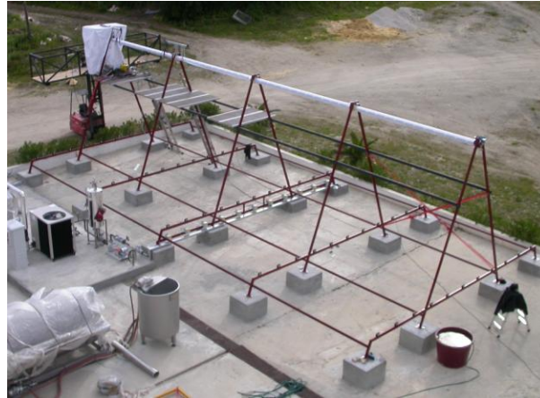
Figure 3-5 The civil foundations and the steel structure of collector during installation.
