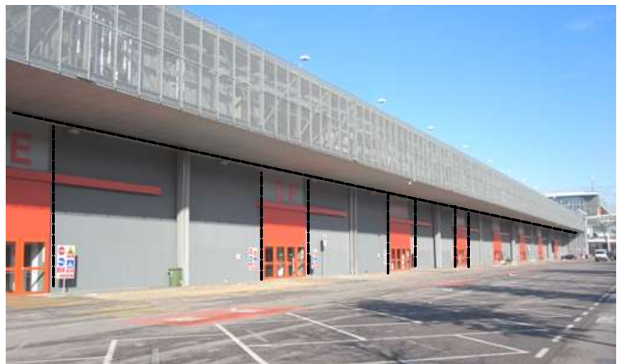
Figure 4-17. Examples of thermal bridges due to the morphology of the building in the representative hall.
