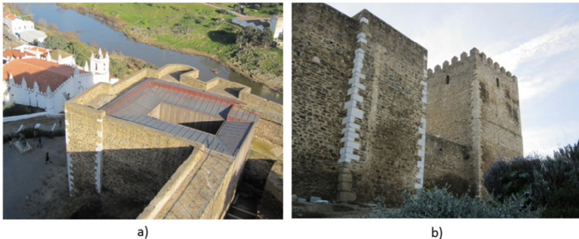
Figure 2.25: Mertula Caslte: the new volume hosting the museum was realized by wooden walls and covered with PVC panels, maintaining it under the skyline of the existing towers (pictures by the author).
