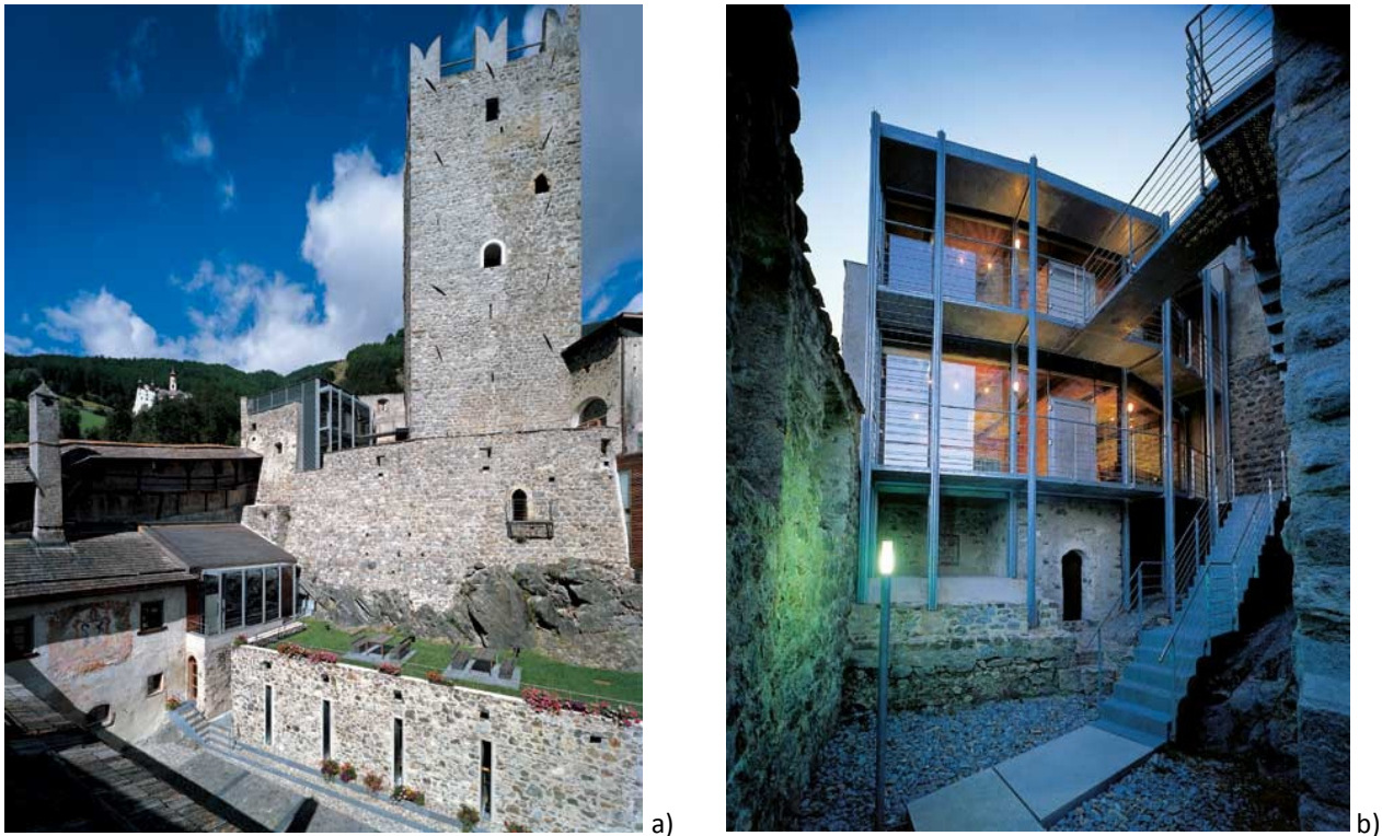
Figure 5.60: Furstemburg Castle: a) view of the partially collapsed tower with the new additions and b) view of the new horizontal and vertical connections (pictures from W. Tscholl's official web site: www.werner-tscholl.com ).
