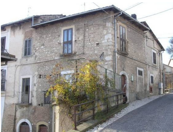
Figure 2.8: Bazzano (L'Aquila). Comparison between two historical buildings stroke by the 2009 earthquake: a) view of an existing building (an aggregate) that was able to face properly to the earthquake; b) view of a collapsed existing building, placed in the nearest of the previous one, that was not able to contrast the seismic actions (author's pictures).
