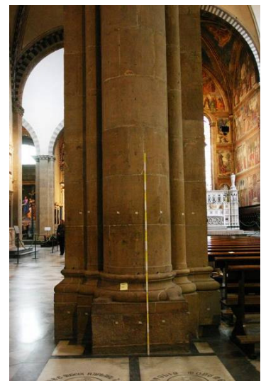
c) south side of pillar P3w
