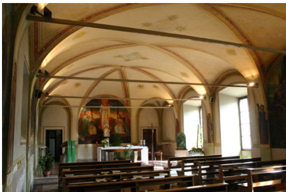
Figure 5.12: Chapel of the convent, covered by a vault built in a style diffused in XV century (author's picture).
