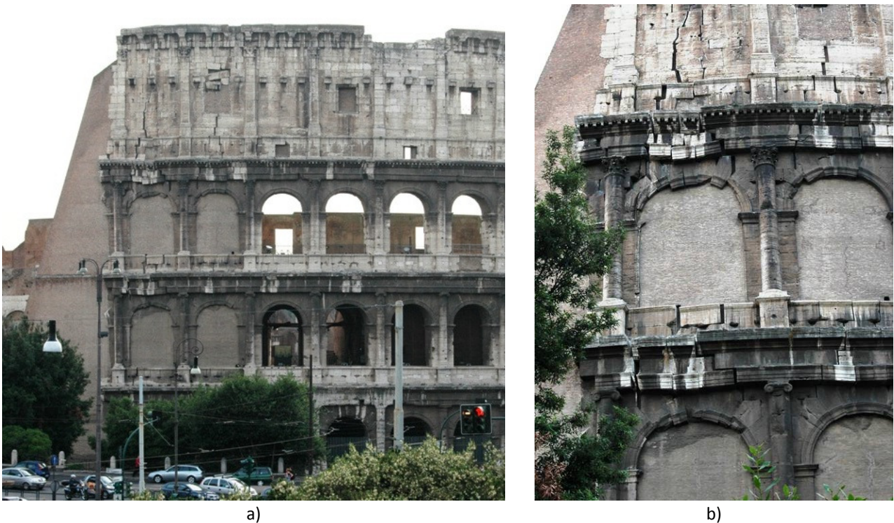
Figure 1.2: View of the Stern's buttress a) incorporating two spans of the external ring of the Coliseum and b) detailed view of the shattered arches blocked in a sort of snapshot of the history (pictures of the author).
