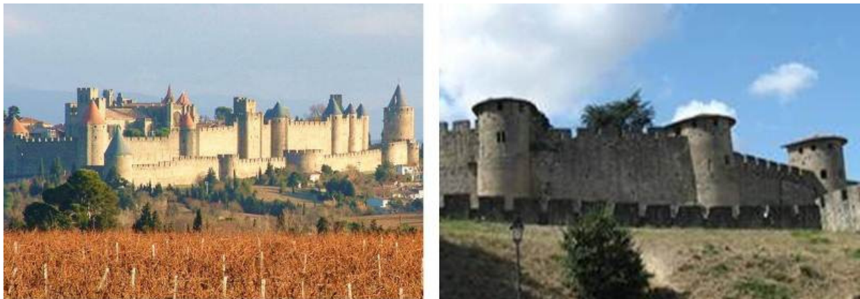
Figure 1.8: Two views of Carcassonne. On the left the defensive walls present the conic roofing design by Viollet le Duc. On the right the conic roofing has been dismantled (pictures free available from the Carcassonne City hall website).
