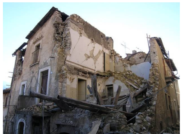
Figure 2.8: Bazzano (L'Aquila). Comparison between two historical buildings stroke by the 2009 earthquake: a) view of an existing building (an aggregate) that was able to face properly to the earthquake; b) view of a collapsed existing building, placed in the nearest of the previous one, that was not able to contrast the seismic actions (author's pictures).
