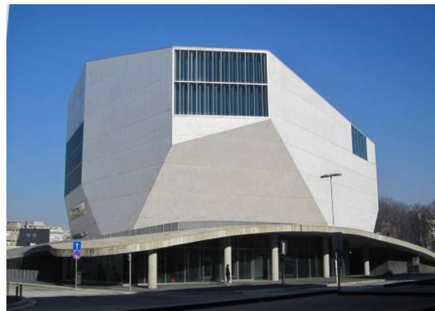
Figure 5.4: view of the Casa da Musica in Porto, designed by R. Koolhaas and realized near the historical centre (author's picture).
