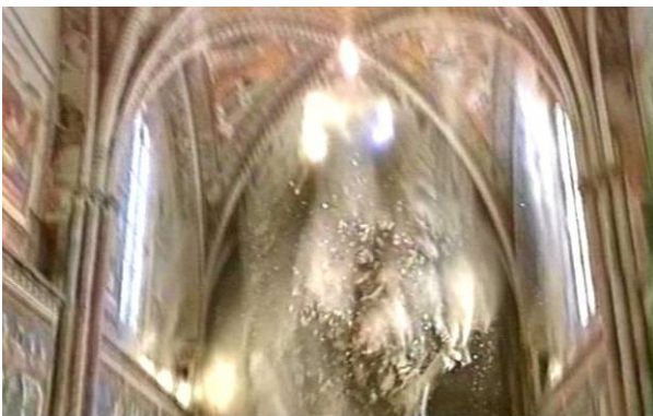
Figure 2.4: Two frames of the video recorded in the superior Basilica of Assisi during the collapse of the vaults of the first two spans of the nave (pictures available in the web at the following link: )
