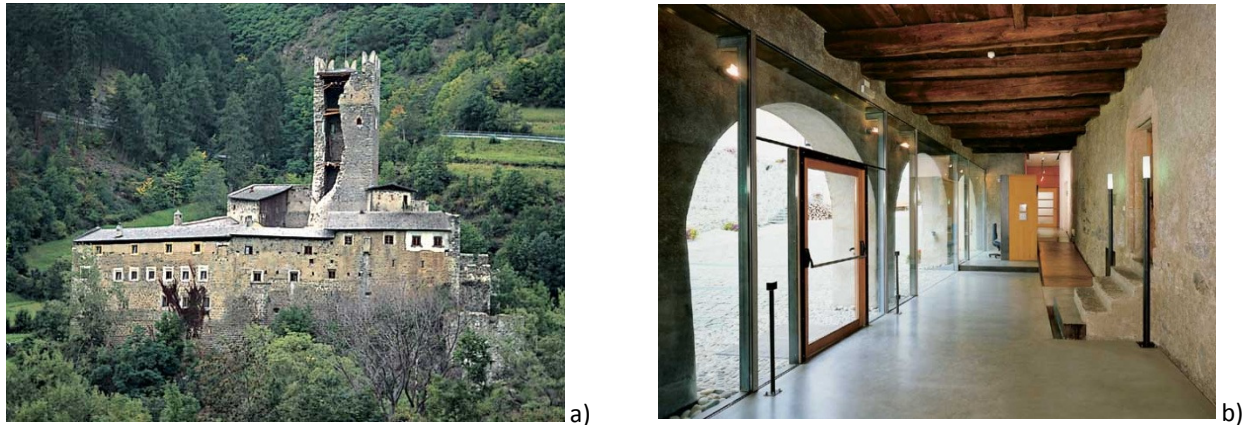
Figure 5.59: Furstemburg Castle: a) view of the partially collapsed tower and b) view of a closed cloister (pictures from W. Tscholl's official web site: www.werner-tscholl.com ).
