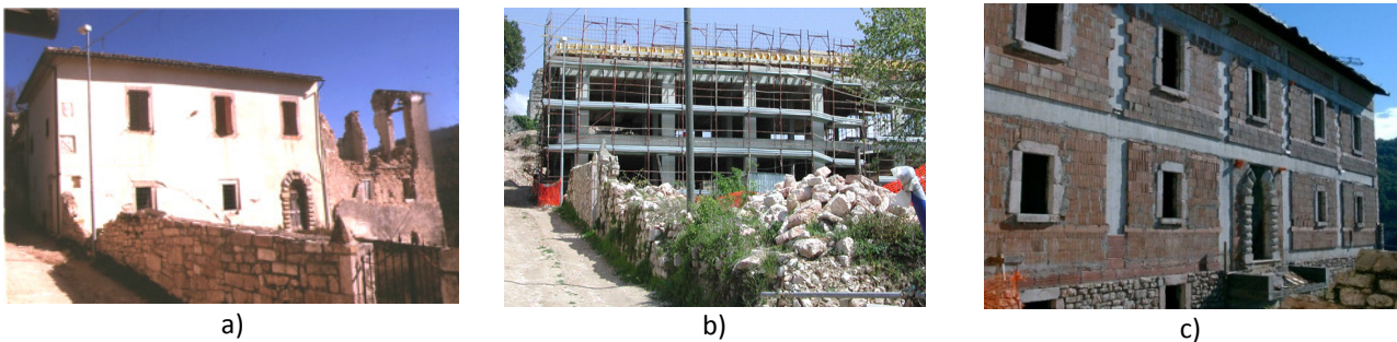
Figure 5.56: Sequence of the reconstruction of a palace stroke by the 1997 Umbria and Marche earthquake: a) 1998 picture showing the conditions of the palace after the earthquake; b) 2002 picture showing the building technology used for the reconstruction (courtesy of arch. A. Saisi); c) 2003 picture showing the modern hollow brick infill between the r.c. structure (picture by the author).
