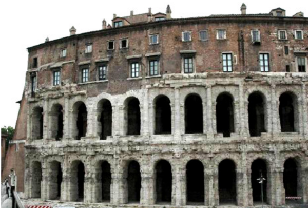
Figure 1.16: View of the Marcello's Theatre in Rome (author's picture).
