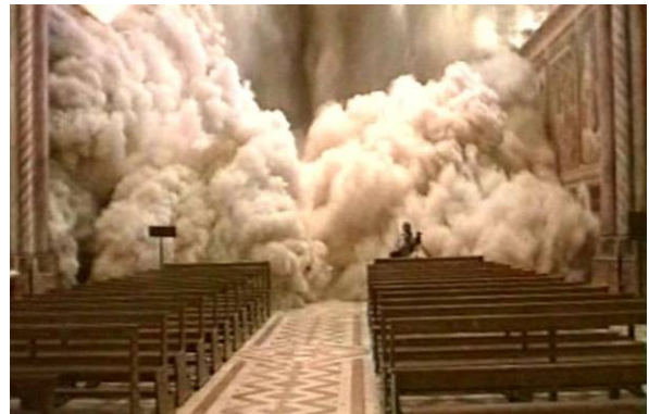
Figure 2.4: Two frames of the video recorded in the superior Basilica of Assisi during the collapse of the vaults of the first two spans of the nave (pictures available in the web at the following link: )
