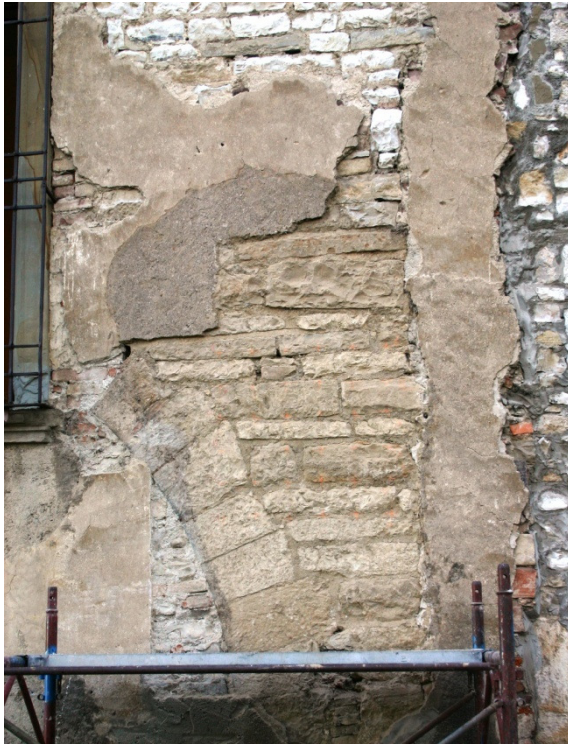
Figure 5.10: Different textures appearing from the decayed plasters on the east façade (author's picture)
