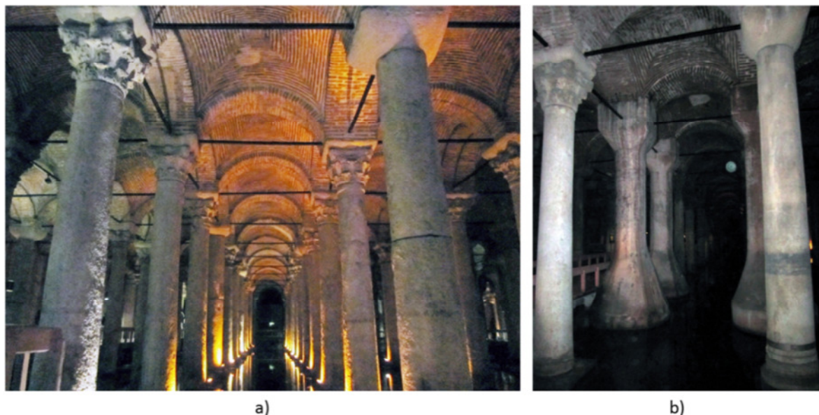
Figure 2.26: a) view of the Roman cistern in Istanbul; b) view of some rebuilt columns and pulvino realized by reinforced concrete (pictures of the author).
