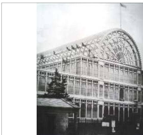
Figura 89 - Crystal Palace, Londra, J. Paxton, 1851 (da SAINT, Architect and Engineer. A Study in Sibling Rivalry , Yale University, 2007, p. 132).
