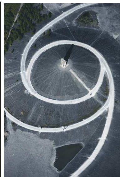
Figure 1.59 The spiral hill, or so-called "stairway to heaven" by Herman Prigann, in Ruhrgebiet, Germany (1998-2005); an example of an industrial spoil; the artificial hill raises 1220m high, with a tower constructed from reclaimed concrete blocks.
