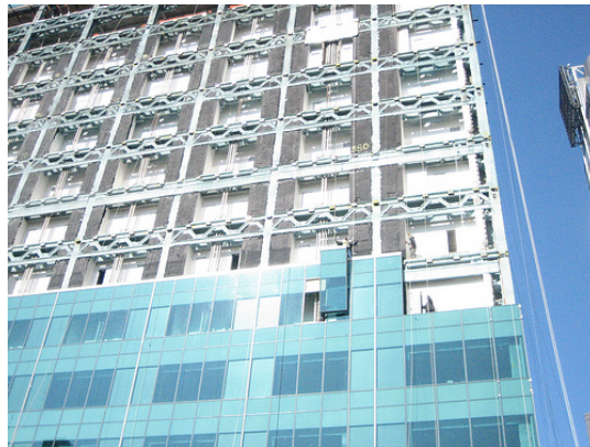
Figure 9: Unitized curtain wall systems
