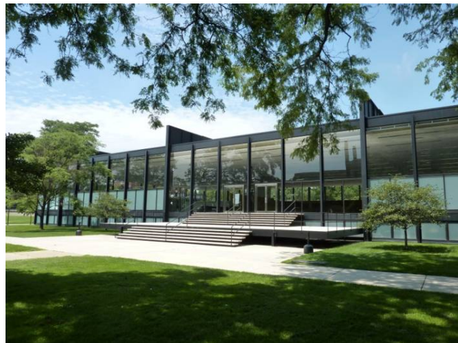
(a) (b) Figure 7: a) Stick system curtain walling; b) IIT Crown hall Mies van der Rohe, 1940
