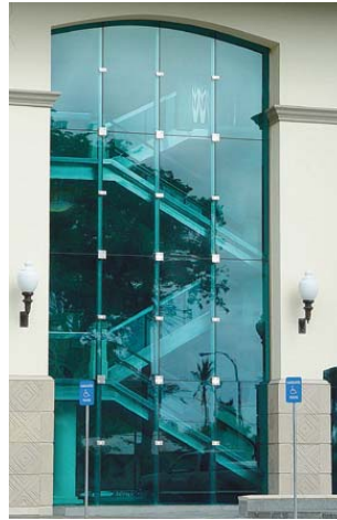
Figure 14: suspended structural glazing
