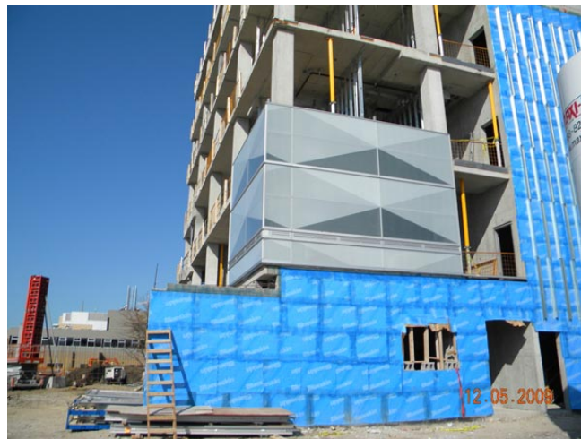
Figure 10: Panelized curtain wall systems
