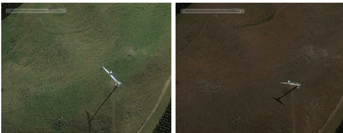
Figure 5.5. Before (09/03/2010, left-hand side) and after (23/02/2011, right-hand side) earthquake satellite pictures of the 500 kilowatt wind turbine located at Gebbies Pass, around 15 km south west of the epicentre of the 22 February Christchurch earthquake. The two pictures show the good seismic response of the structure.
