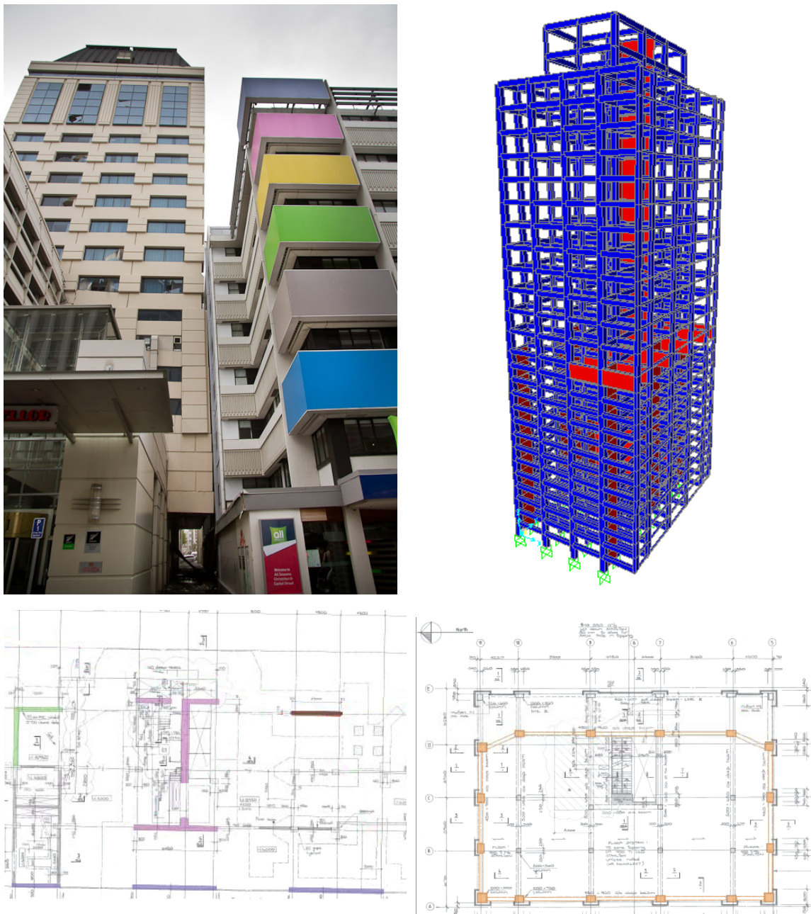
Figure 5.13. Top: Picture of the Grand Chancellor Hotel in the Christchurch CBD, after the earthquake (left hand side) and its numerical model with FE code (right hand side). Bottom: Technical drawing of a typical building story, from level 1 to 14 (left hand side) and from level 15 to 28 (right hand side).
