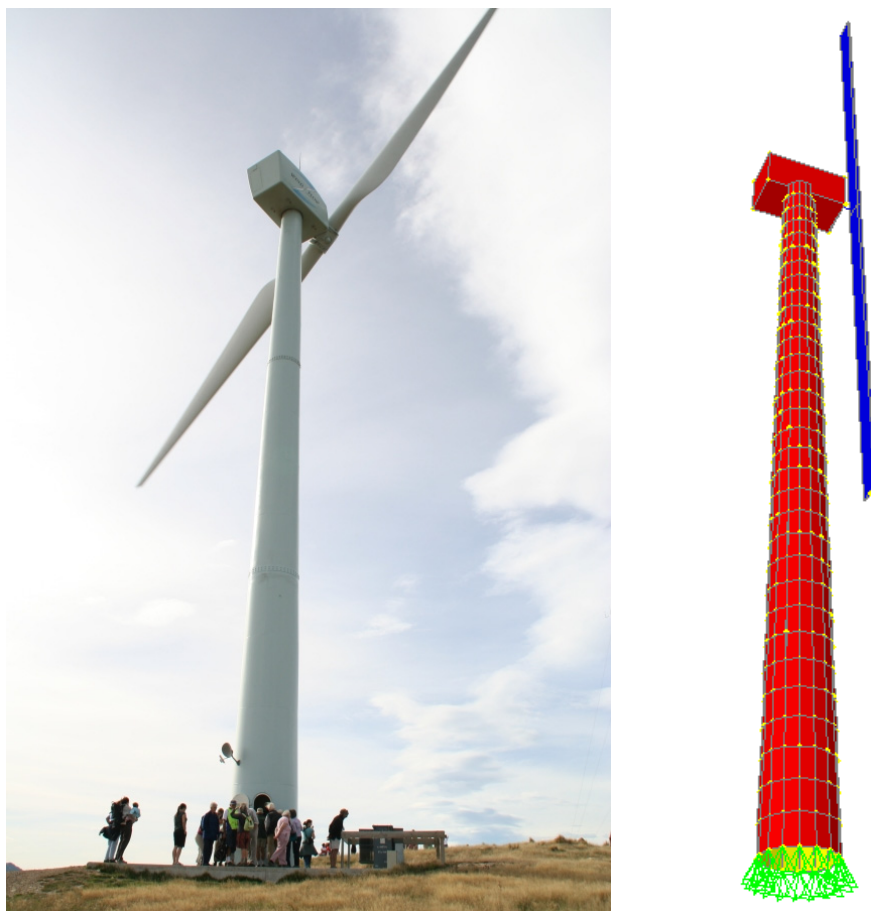
Figure 5.9. Picture of the Wind tower installed at Gebbie Pass (left hand side) and its numerical representation with FE code (right hand side).
