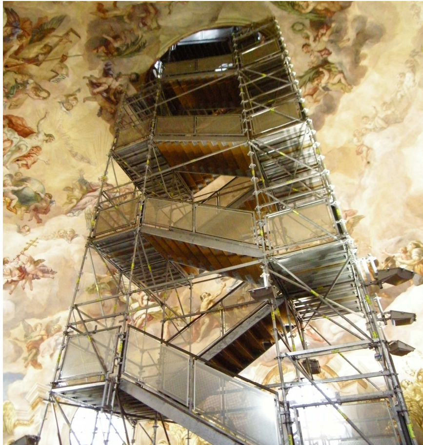
Figure 23: Scaffolding in St. Karl Borromäus Church, Vienna.
