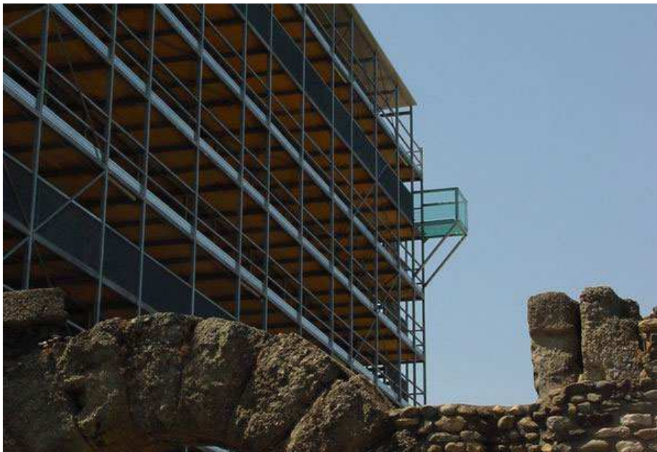
Figure 22: Scaffolding at the Aosta Roma Theater
