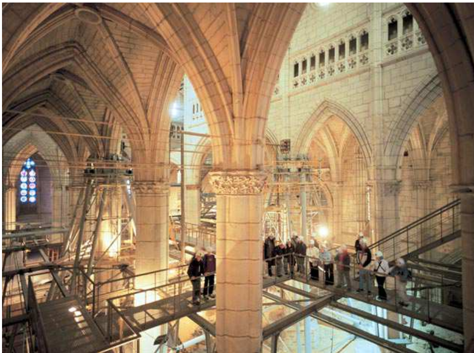
Figure 24: Scaffolding open to public in Cathedral of Santa María de Vitoria.
