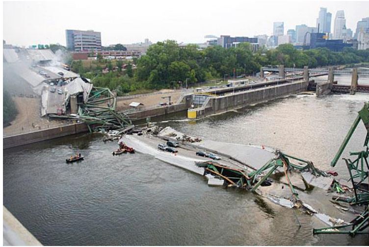
Figure 1-1: August 1, 2007 Minneapolis I-35W highway bridge collapse
