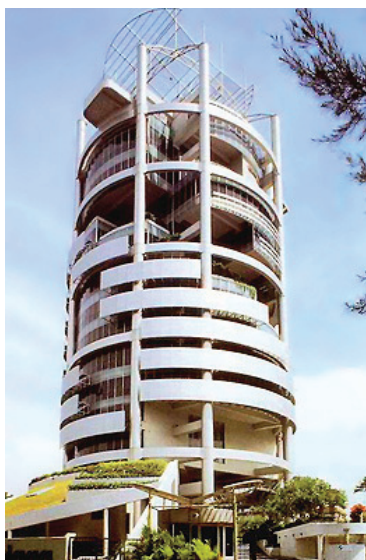
Ken Yeang Menara Mesiniaga Tower, Subang Jaya Selangor, 1992
