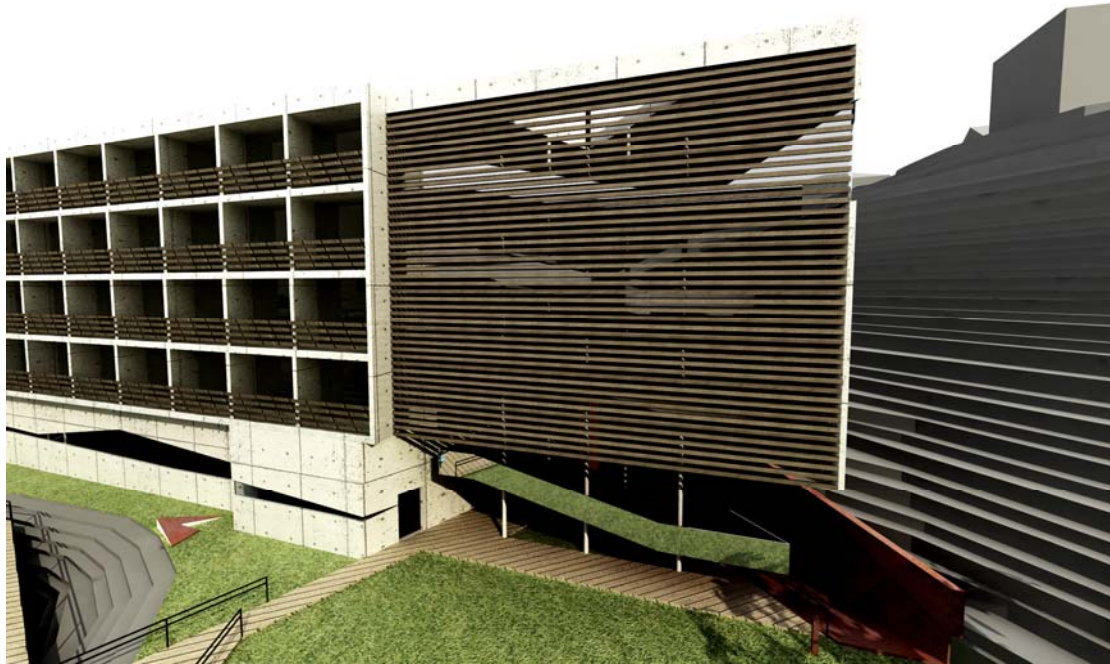
Figure 3.25 Facade of Semi-Enveloped courtyard
