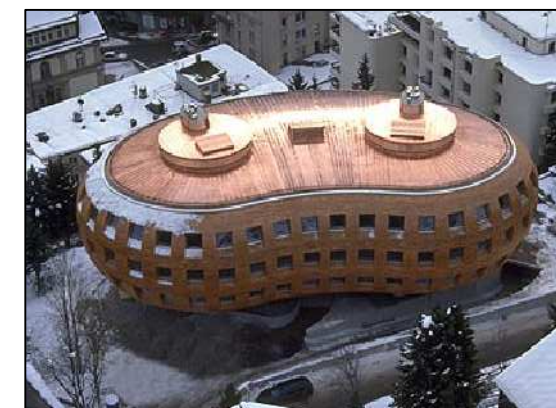
Vista aerea (googleimages.com)
