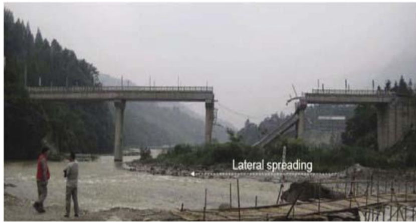
Figure 1.9. Gaoyuan Bridge nearby fault trace, 2008 Wenchuan earthquake [11]
