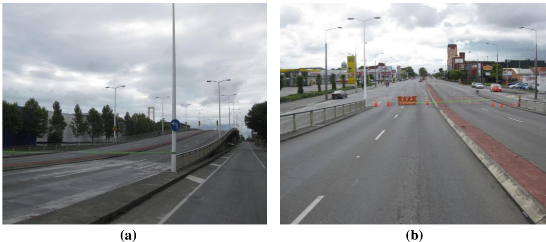
Figure 6.12. View of the bridge (a) from the west side and (b) from the east side.
