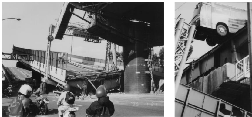
Figure 1.4. Example of collapsed span as a result of insufficient support length, 1995 Kobe earthquake [10]
