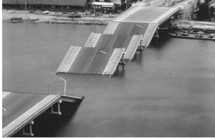
Figure 1.1. Showa Bridge collapse in 1964 Niigata earthquake.
