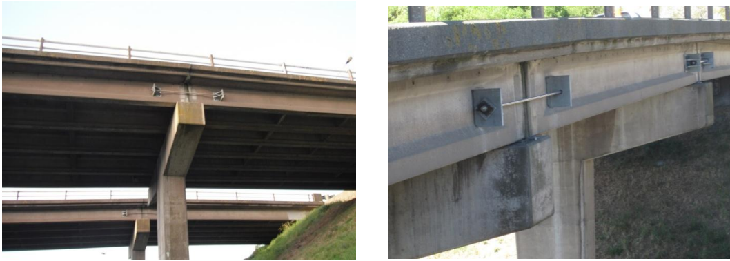
Figure 5.2. Steel linkages between spans after the retrofit program.
