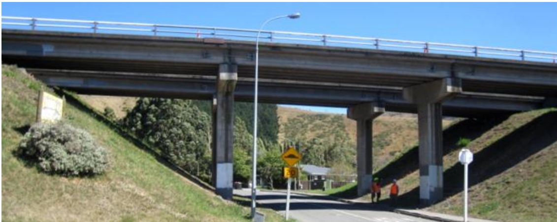
Figure 5.1. Overall view of Horotane Valley Overpass.
