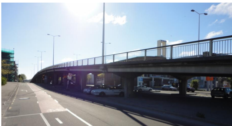
Figure 6.1. View from South-West of Moorhouse Overbridge [A. Palermo].
