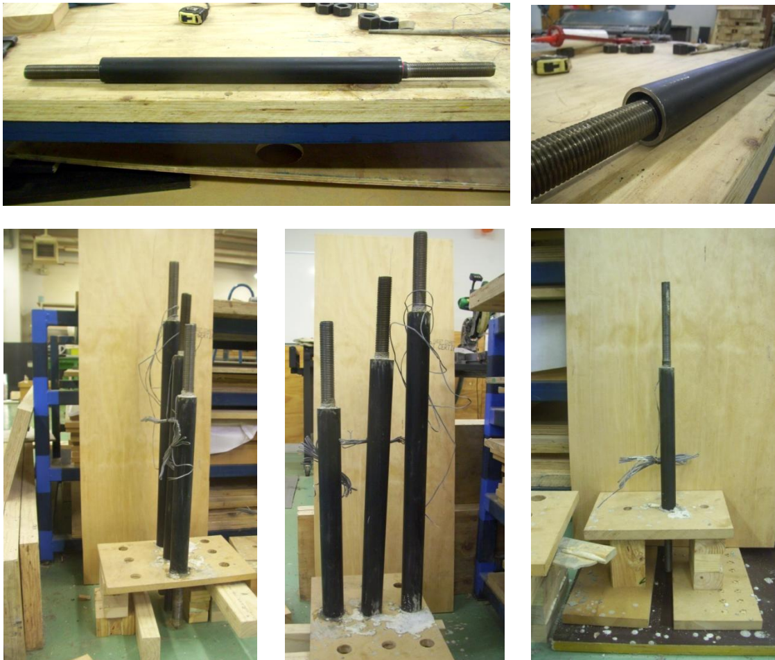
Figure 90. Manufacturing of External “Plug and Play” Dissipators
