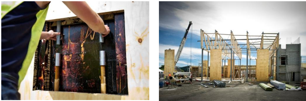
Figure 185. Macalloy Bar Connection (left); Construction Progress (right)
