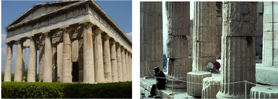
Figure 22. Earlier implementation of a self-centering limited-damage rocking system, for earthquake loading (Dionysus temple in Athen [2])
