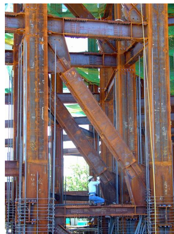
Figure 15. Components of BRB (left); Example of BRB of the Tzu-Chi Culture Building (Taipei, Taiwan) [5]
