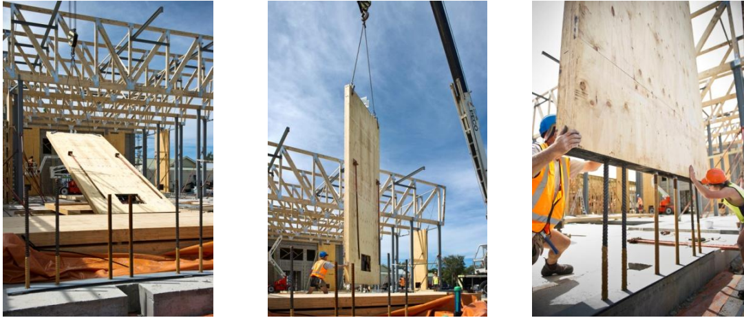
Figure 184. Wall Panel Erection
