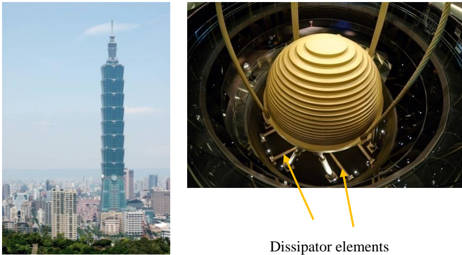
Figure 21. The Taipei 101, Taiwan (left); the Tuned Mass Damper (right) http://en.wikipedia.org/wiki/File:Taipei_101_Tuned_Mass_Damper_2010.jpg
