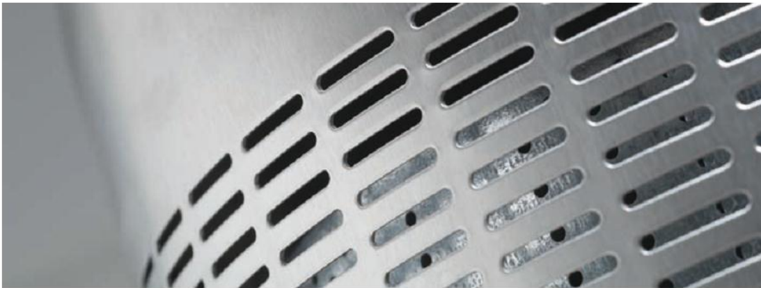
Figure 193 A closer look to a diffuser
