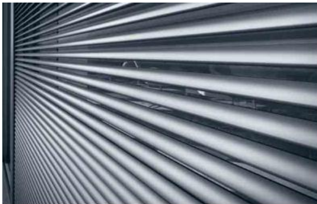
Figure 145 E2 facade with shading
