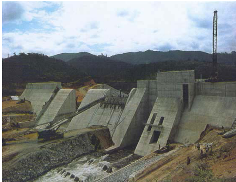
Figure 4.20.: Lower Kihansi dam
