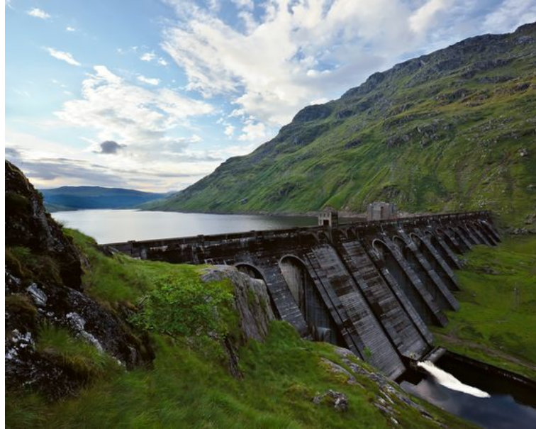
Figure 7.2.: Buttress dam
