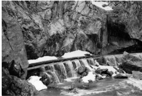
Figure 7.13.: Lateral spillway
