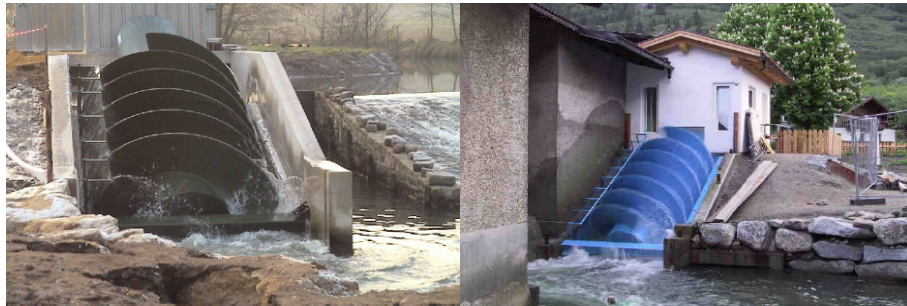
Figure 8.9.: Cochlea screws
