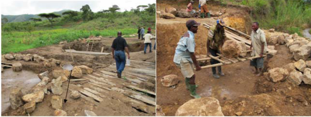
Figure 22.8.: Macheke, bridge construction
