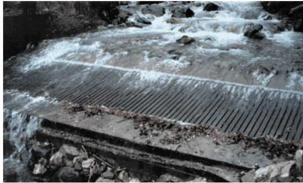
Figure 7.10.: Drop intake
