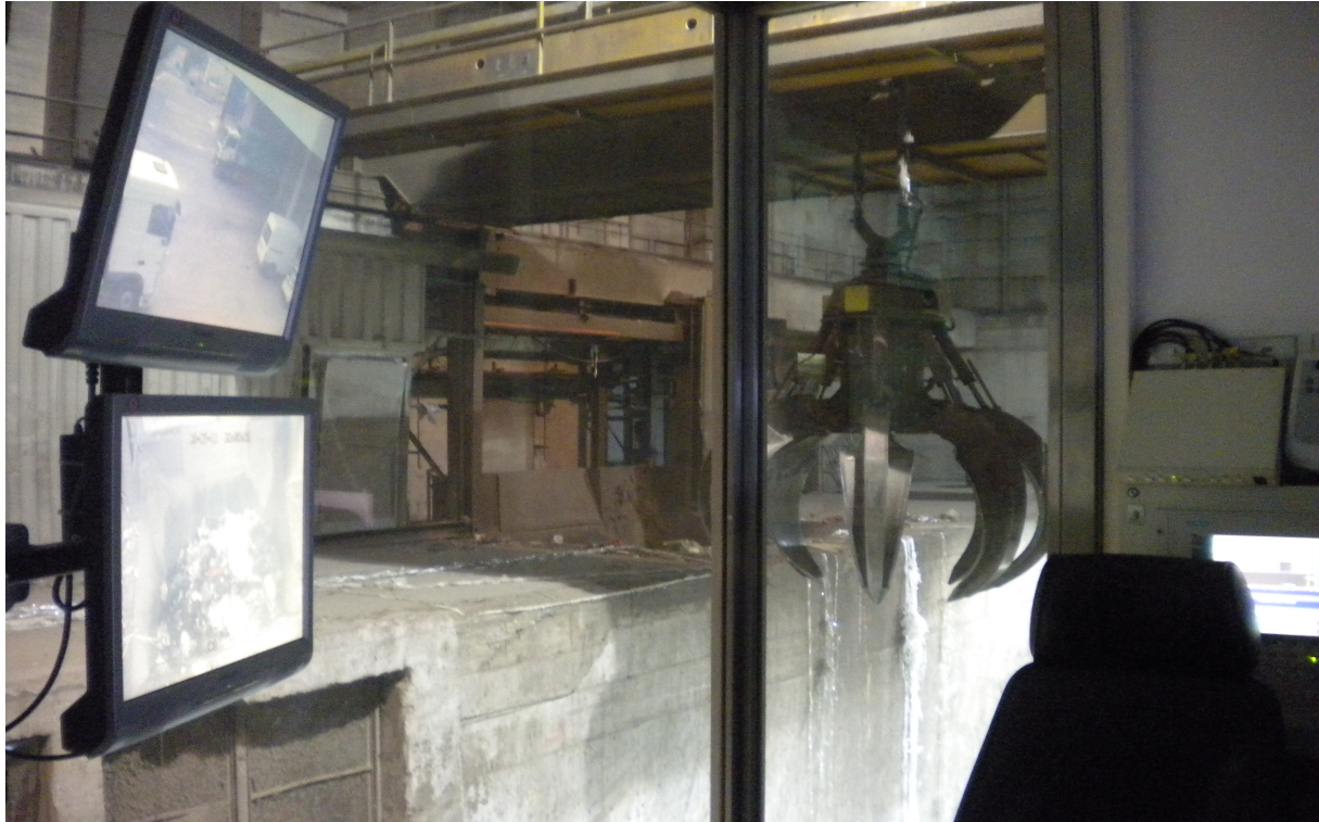
Figure 2.3.4 - Doped waste charge preparation: after the second mixing performed through the waste grab, the doped waste is ready to be introduced into the feeding hopper of Valmadrera WTE plant.
