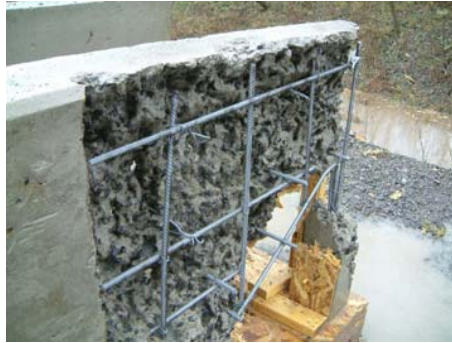
Figure 2.15.: Steel rebar after water jet fragmentation
