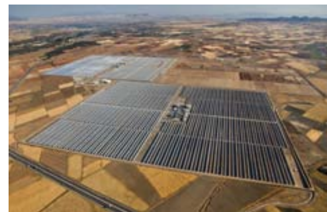
Andasol Solar Power Station Aproximately 200 ha Andalusia, Spain
