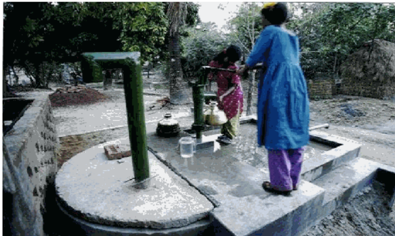
Picture-3.1: Water collection from a closed dug well by tube well (74)
