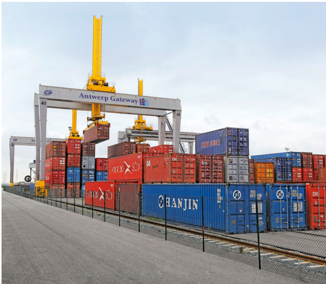
Figure 9 – A fully Automated Stacking Crane, operating in Belgium
