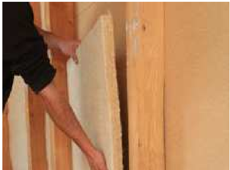
Fig. 1.18 Posa matterassini Technichvre Hempwool
