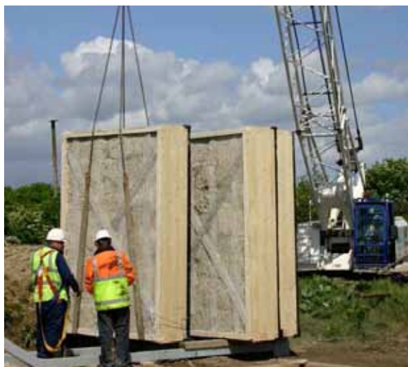
Fig. 3.215 Pannelli strutturali, Modcell, www.modcell.com
