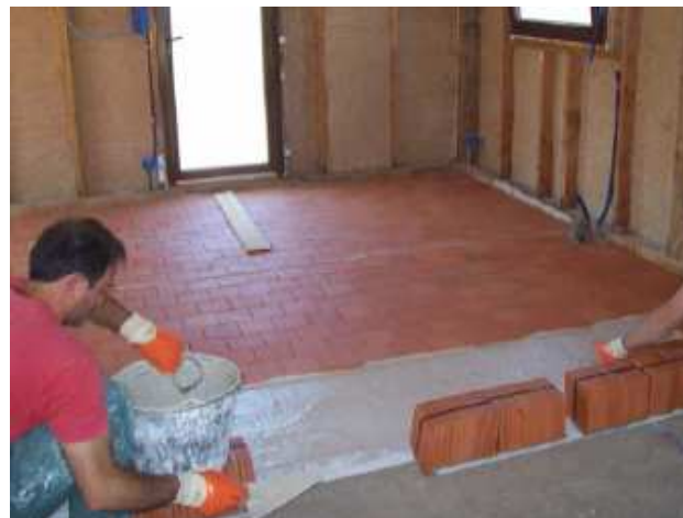
Fig. 3.96 Posa delle piastrelle da Technichanvre, Cahier_techniques_DALLAGE, www.technichanvre.com
