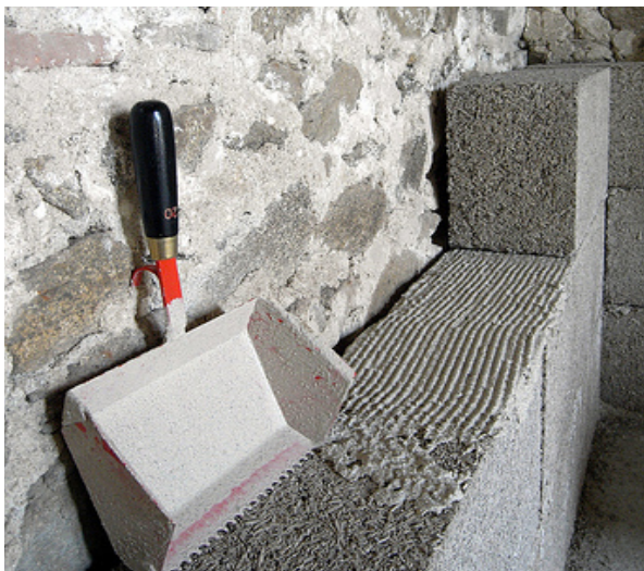
Fig. 3.189 Controparete in blocchi Chanvribloc, www.chanvribloc.com/Isolation int
