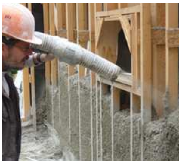
fig. 3.155 Muratura a spruzzo, INATER www.inater.net
