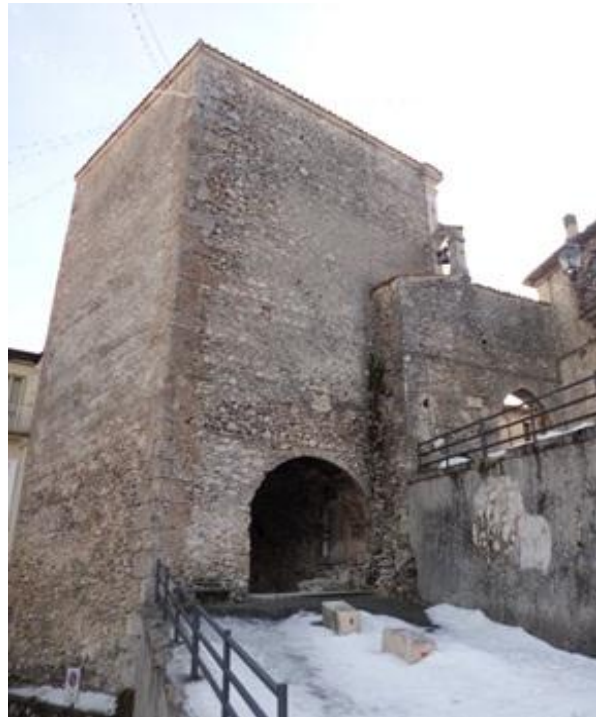
2.37 Front North-West Façade (Aggregate CdM Tower)
