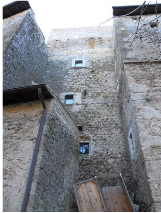
Figure 3.7 SSS 017 Front North
