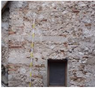
2.21 Tower House – Masonry 1 – Photo
