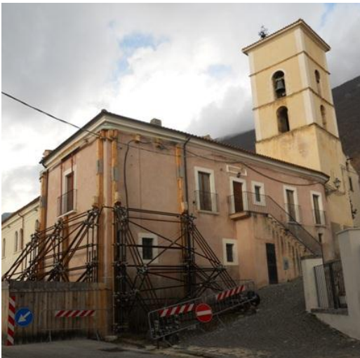
Figure 5.6 Church of Aggregate VSL 012
