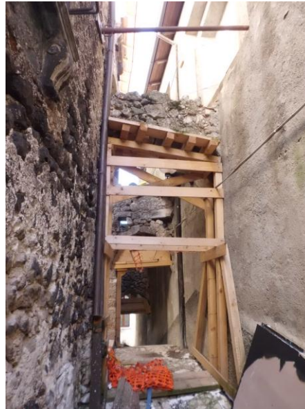
Figure 3.123 Opening Support
