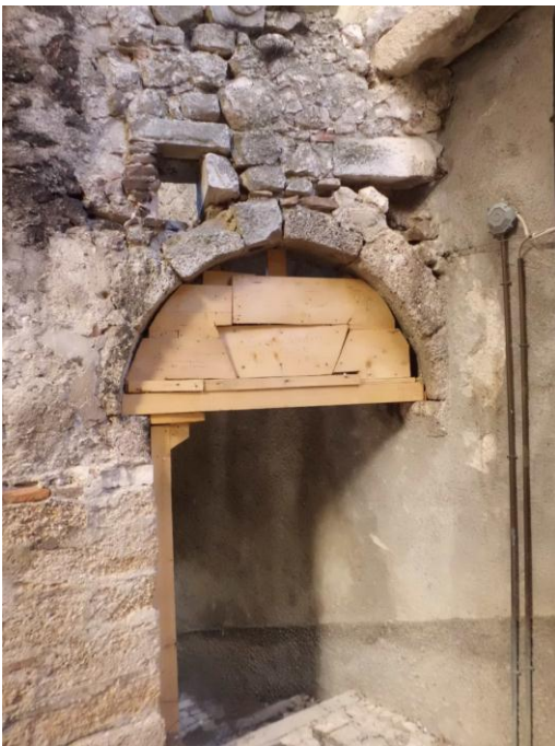
Figure 3.121 Arch Support Intervention
