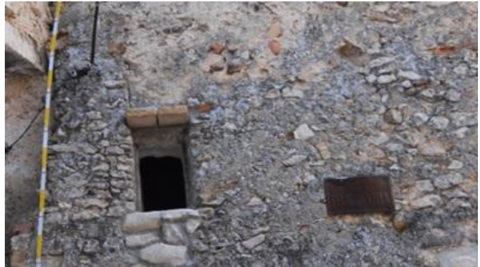
Figure 2.15 Masonry Elevation – Typology 2 – Elevation
