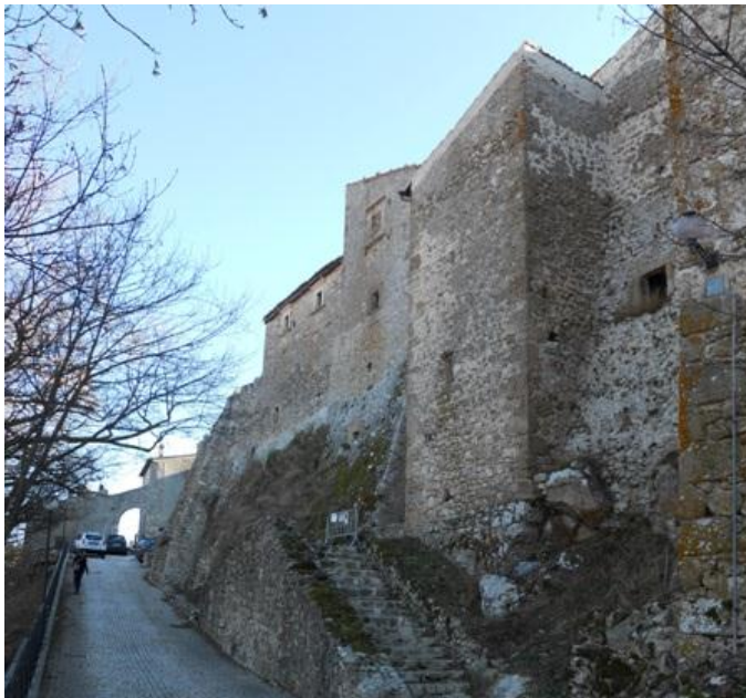
Figure 3.4 Aggregate SSS 013 Front North
