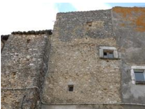
2.19 Front-North Façade (Aggregate CdM 031)
