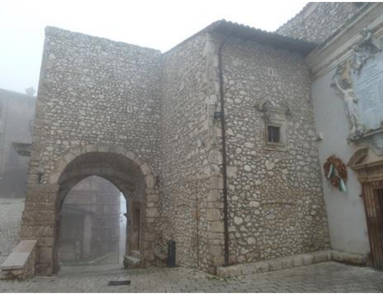
Figure 3.15 SSS 047 Front East
