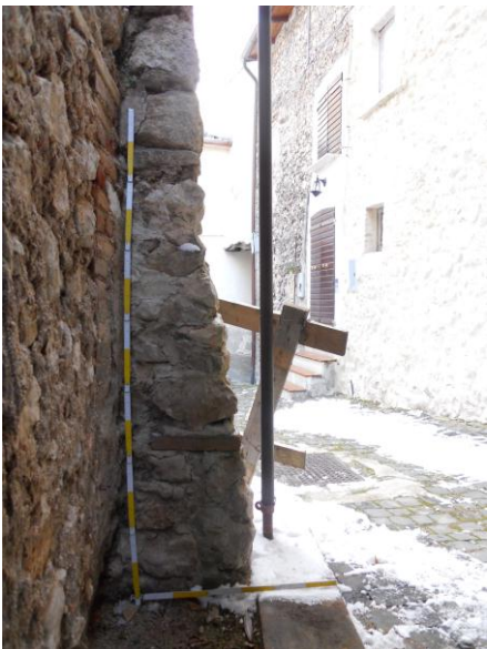
Figure 5.98 Partial Buttress
