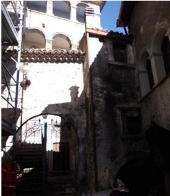
Figure 3.18 SSS 068 Front East
