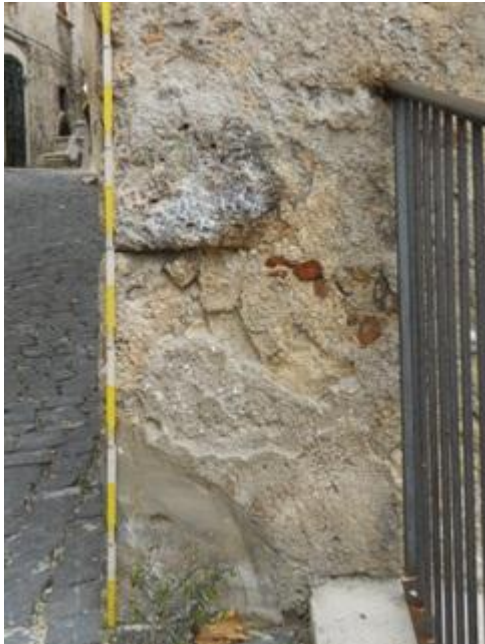
Figure 2.23 Front North Façade
