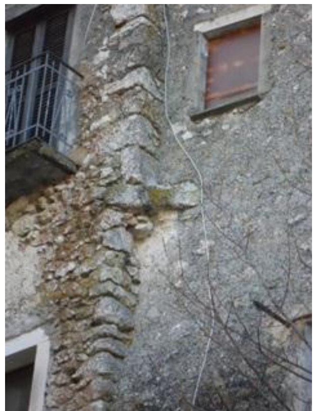
2.20 Front-North Façade (Aggregate CdM 031)
