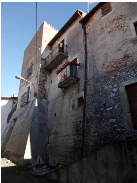
Figure 4.104 Partial Buttress
