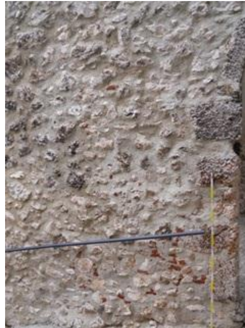
Figure 2.24 Front North Façade
