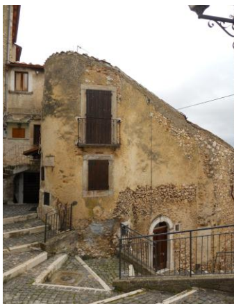
2.109 South-East Elevation of Aggregate
