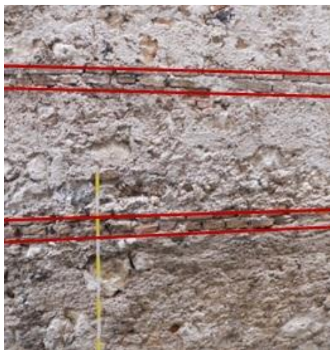
2.31 Masonry Elevation – Typology 2 – Zoom
