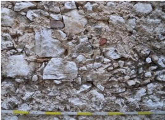
Figure 2.14 Masonry Elevation – Typology 1
