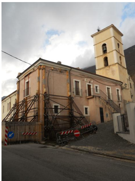
Figure 5.106 Wall Prop Intervention
