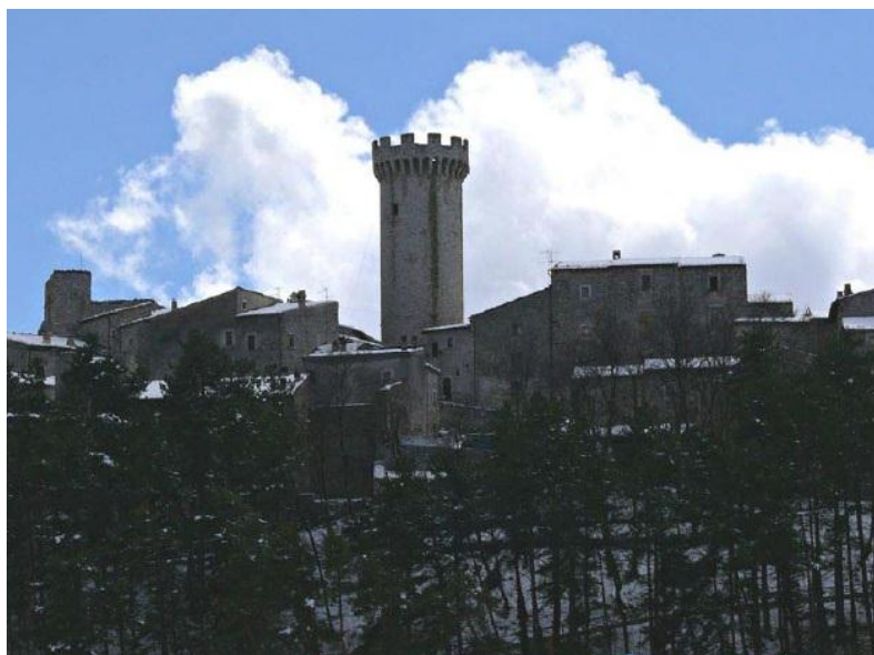
Figure 3.129 Pre-Seismic Medicea Tower
