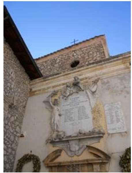
Figure 3.16 SSS 047 Front East
