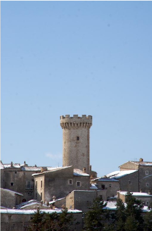
Figure 3.8 Pre-Seismic Medicea Tower
