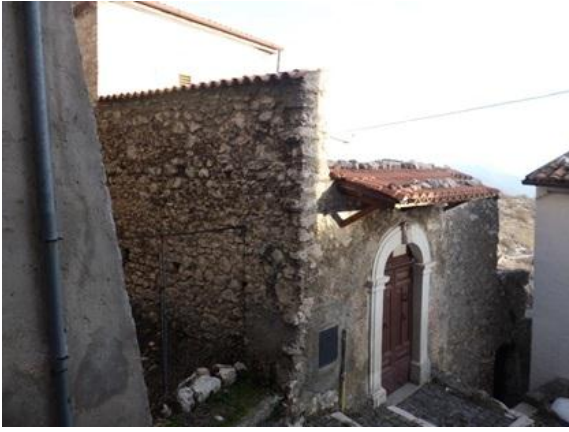
2.43 Front West Façade (Aggregate Cdm 014)
