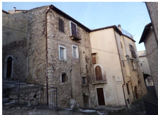
2.110 North-East Elevation of Aggregate
