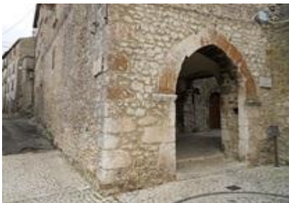
2.36 Front West Façade (Aggregate CdM 010)
