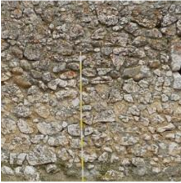
2.38 Parallel Orientation – Masonry 2 – Photo
