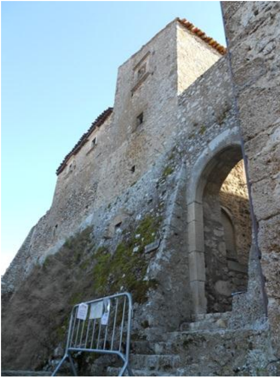
Figure 3.6 Aggregate SSS 013 Front North
