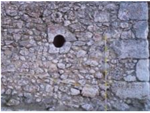
Figure 2.33 Tower- Masonry 2 - Photo
