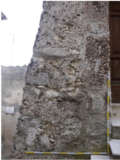
2.130 Example of Buttress in CdM
