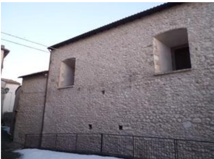
Figure 2.48 North Façade (Aggregate CdM Church 2)
