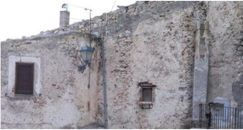
2.30 West Side Façade (Aggregate CdM 001)
