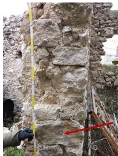
Figure 5.25 VSL 011-A Masonry Section Two
