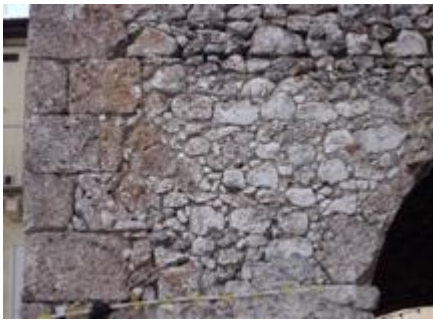
2.35 Front West Façade (Aggregate CdM Tower)
