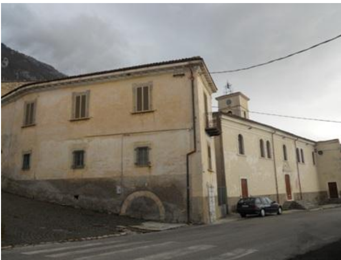
Figure 5.7 Church of Aggregate VSL 012
