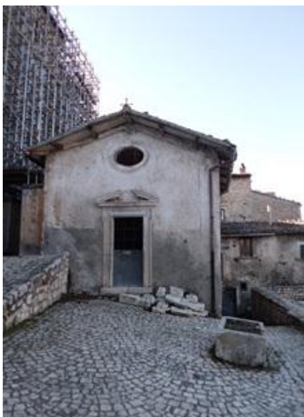
Figure 3.17 SSS 014 Front East
