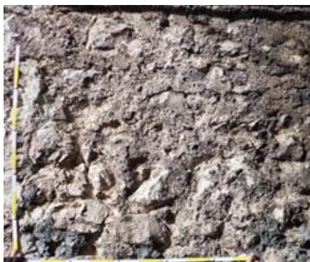
2.25 Parallel Orientation – Masonry 1 – Photo
