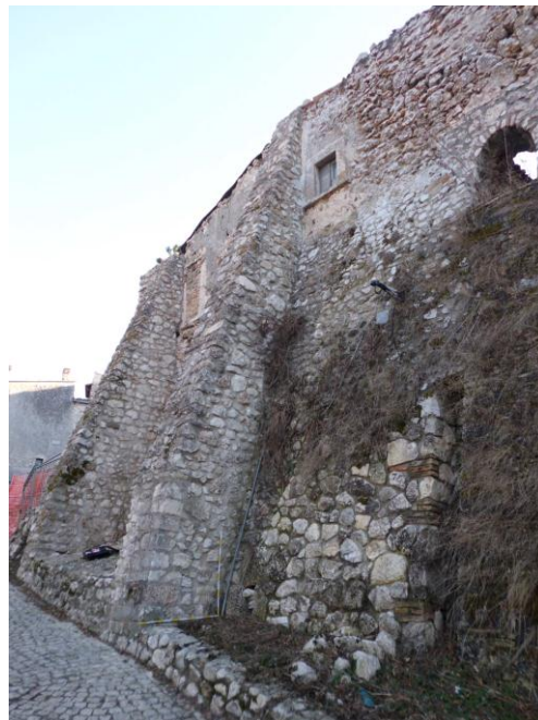
Figure 3.114 Complete Buttress
