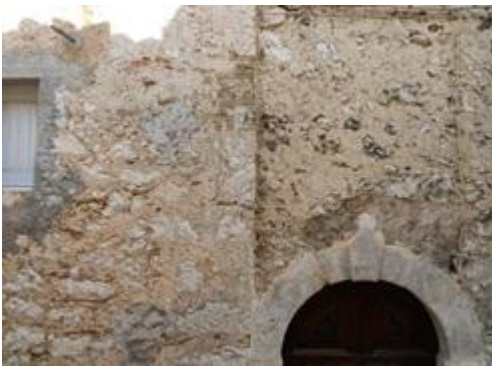
2.18 Front-South Façade (Aggregate CdM 031)
