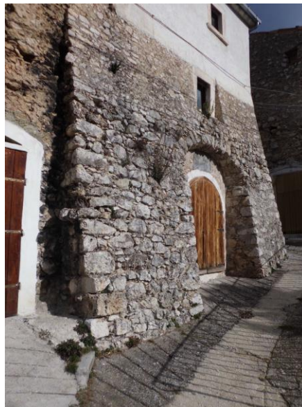
Figure 5.99 Complete Buttress
