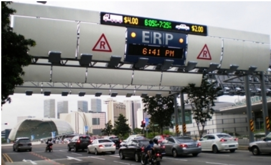
Img.22 Electronic Road Pricing Gantry
