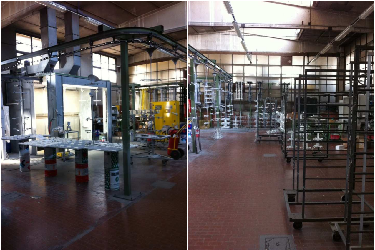
Figure 3.17– Infrastructures and products inside the painting room
