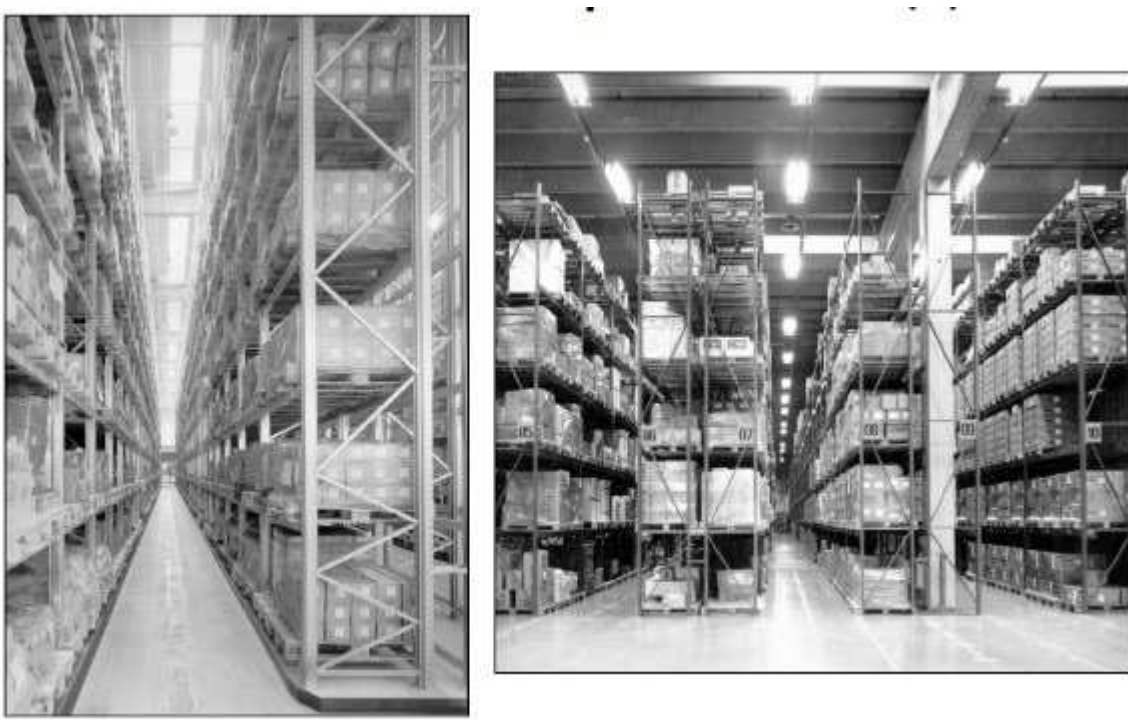
Figure 3.4 - Selective pallet rack system
