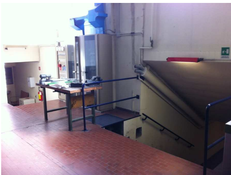
Figure 3.15 - The underground passage between Building 1 & Building 2 .
