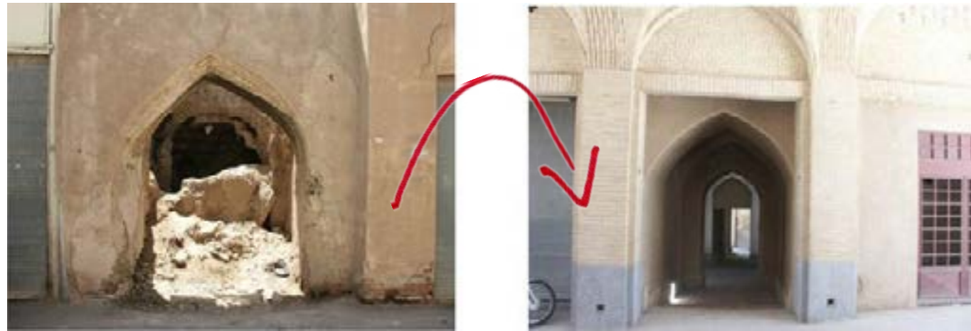
39. restoration of a quarter center in the area: facade and paving restoration-fortifying the structure (source: http://www.imbf.ir )
