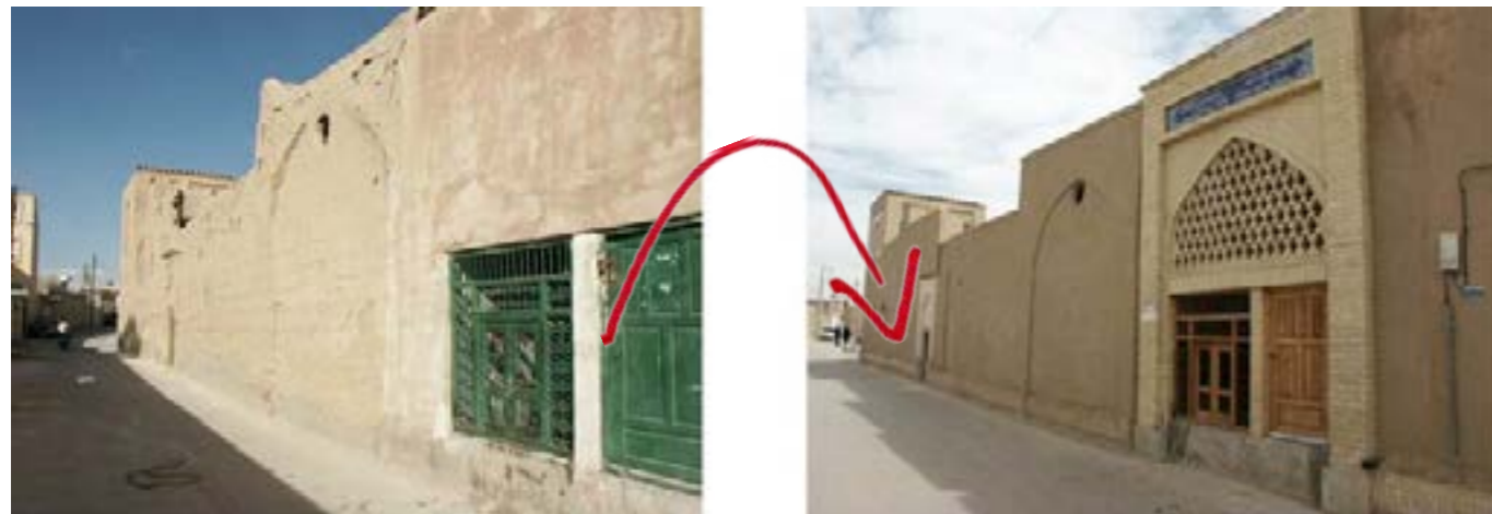
40. restoration of a historical monument: facade and paving restoration-fortifying the structure (source: http://www.imbf.ir )
