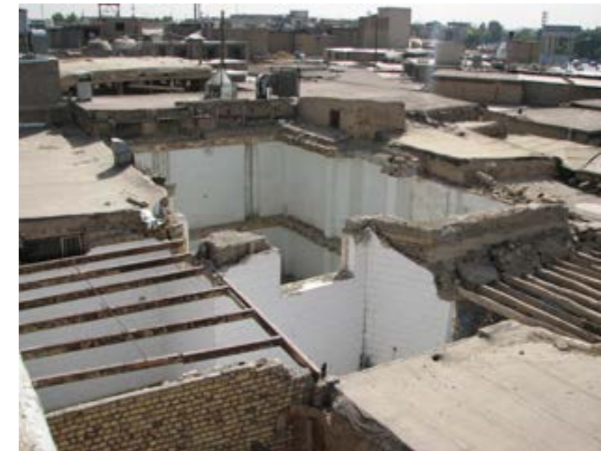
124.The project area’s being in state of decay (source: NAQSH, E, JAHAN-PARS) Consulting Engineers, 2010.)
