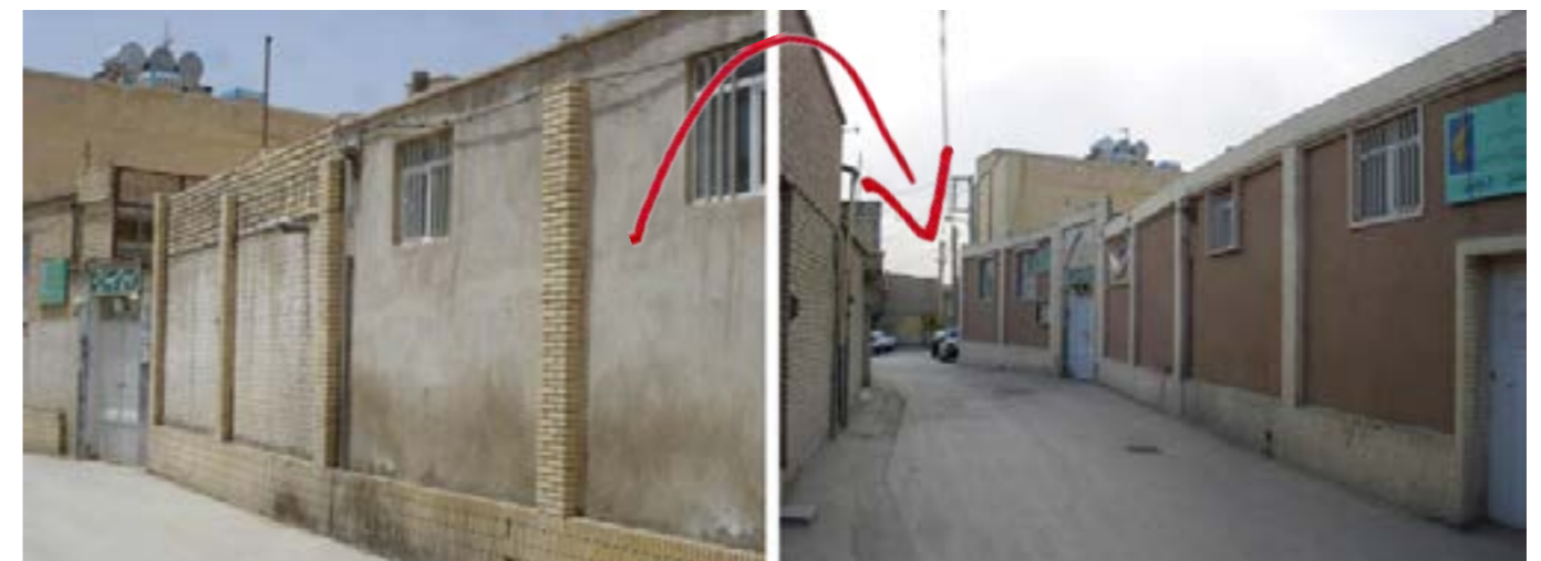
27.facade modification interventions(source: http://www.imbf.ir )
