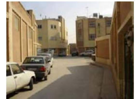
29.restoration of the residential plots (source: http://www.imbf.ir )
