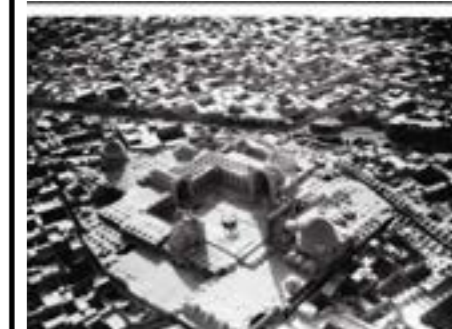
58. The Jameh Mosque of Isfahan (source: NAQSH, E, JAHAN-PARS Consulting Engineers, archive, 2010.)
