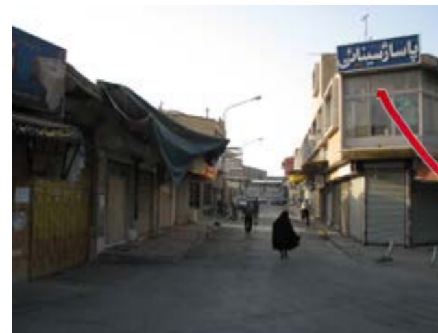
150.a degraded street on Majlissi Street (source:NAQSH, E, JAHAN-PARS) Consulting Engi-neers,2010.)
