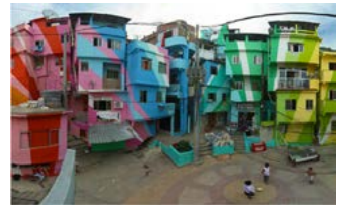
142.improvements of facades:favelas painting Rio De Janeiro in a low class neighborhood in (source:http://www.favelapainting.com/santa-marta)
