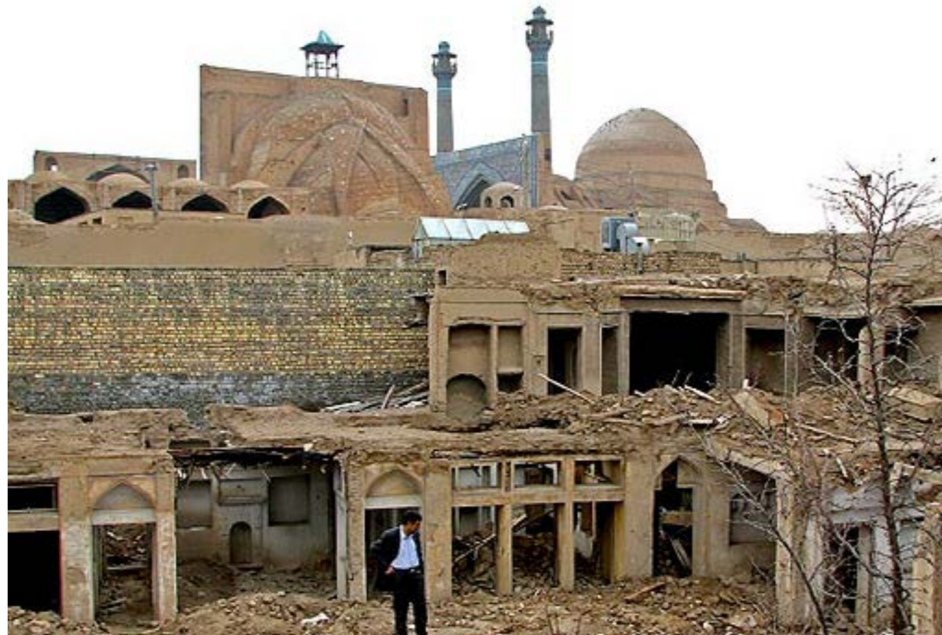
82.Bottom:a blighted plot adjacent to Jameh mosque (source: http://www.mehrnews.com/fa/newsdetail.aspx?NewsID=812331 )
