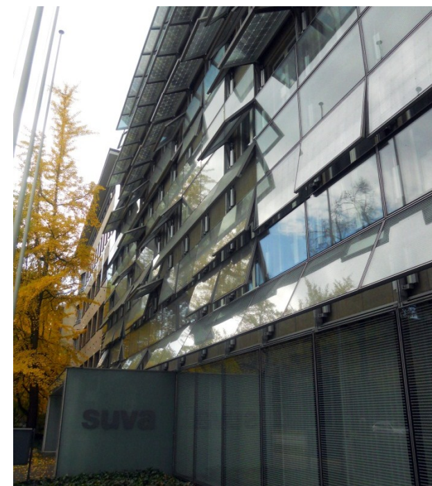
72. SUVA Building. Esterno
