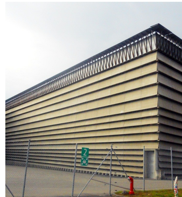
41. Esterno Ricola Storage Building
