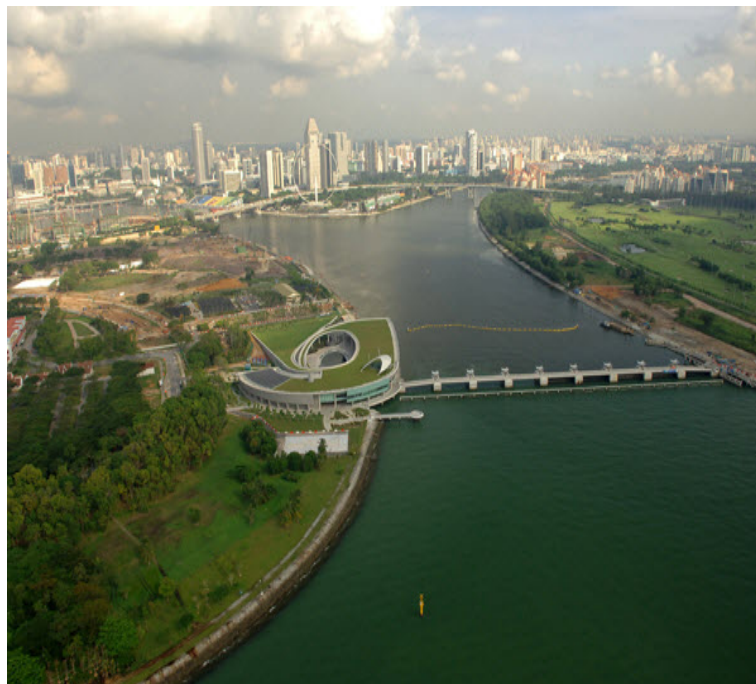
(b) Overview of the Barrage and the visitor center where pumps are located
