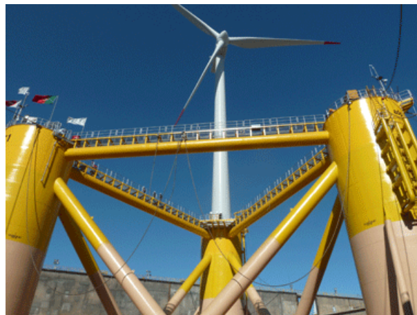
Figure 2.2.: WindFloat semisubmersible structure and 2MW wind turbine.
