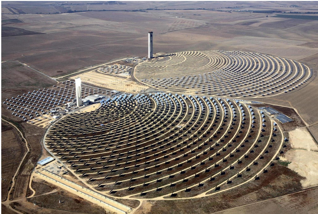
Figure 1.14: Aerial view of the PS10 and PS20 power tower near Seville.
