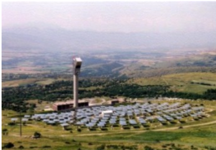
Figure 2.4: Aerial photo of the Themis solar tower.
