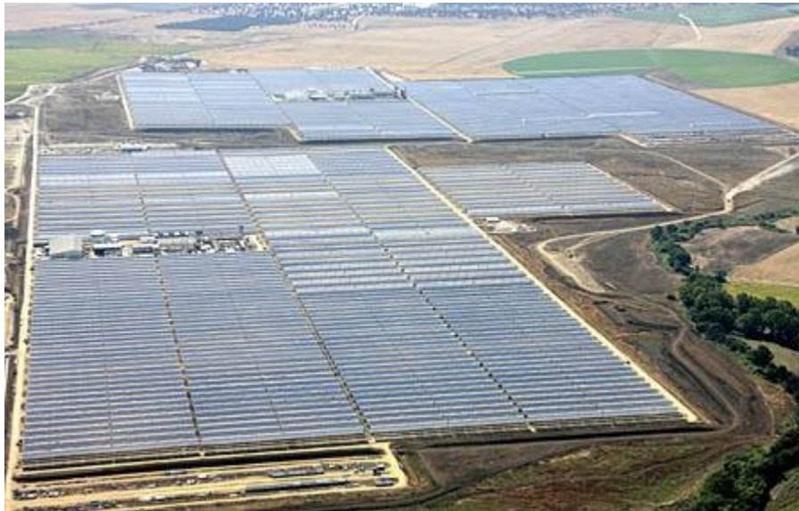
Figure 1.9: Albengoa Solar's Solnova 1 (50 MW e ).
