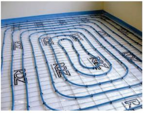
Fig. 5.67 heating wires system
