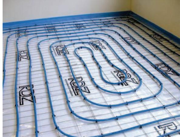
Fig. 5.67 heating wires system
