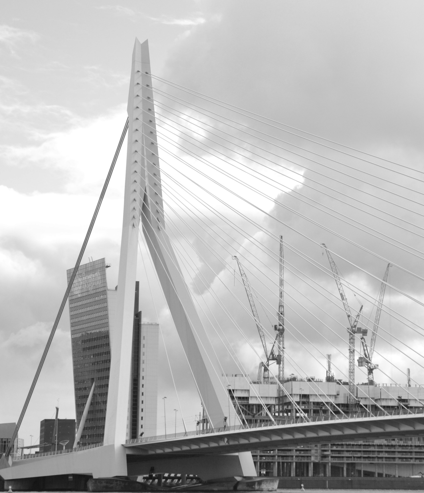
fig. 2 - Erasmus Bridge, Rotterdam
