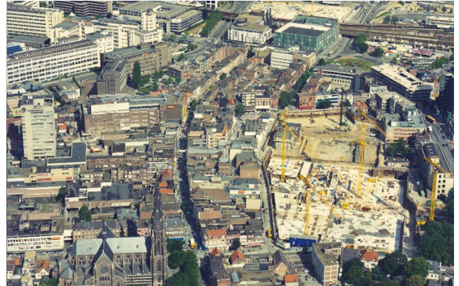
3.1.2 - Construction site and surroundings
