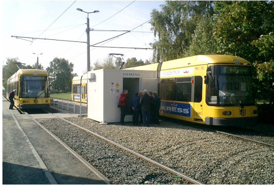
Figure 1.8. Siemens SITRAS SES full time installation in Dresden (Hellerau).
