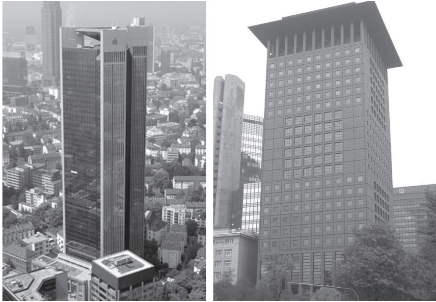
Figure 3.4: Trianon and Taunustor building, Frankfurt
