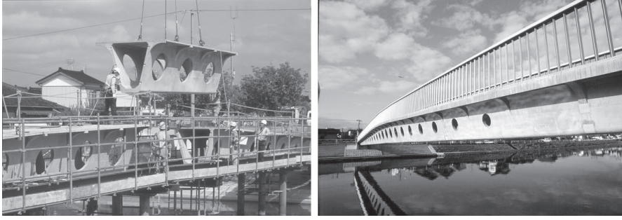
Figure 3.2: Sakata-Mirai Footbridge, Japan, 2004
