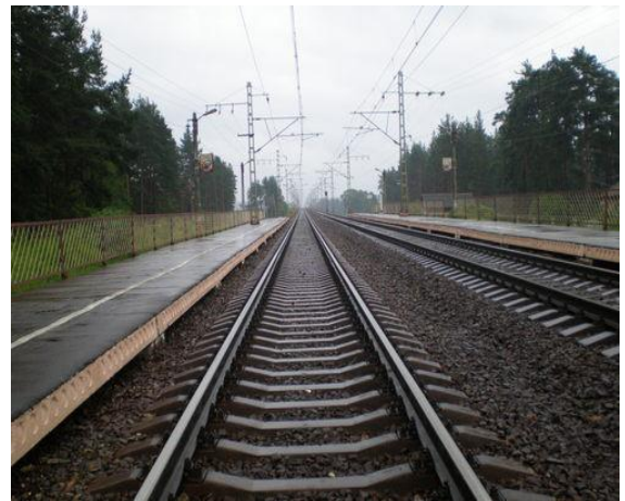
Figure 2.8. Railway station «Tvertsa»
