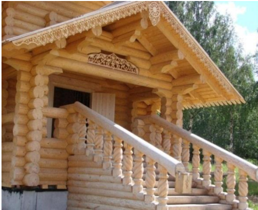
Figure 2.130. Wooden house decorations
