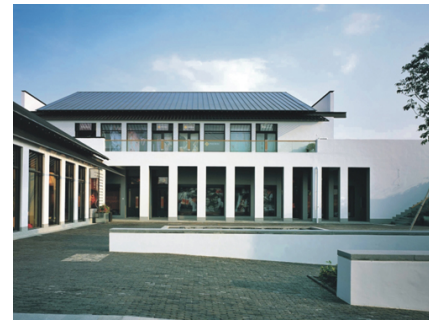
3.3 Various space in Chinese Residence
