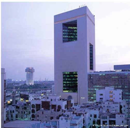
5.28 Building from the city
