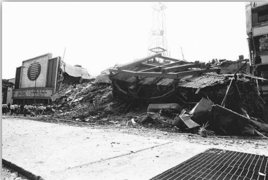
Figure 15 The collapsed transmission tower of Televisa [14]
