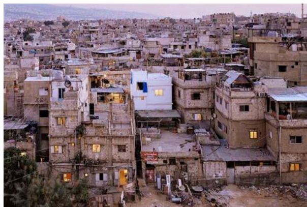
Photo 4-3: Two additional floors are visible on the building in the bottom left corner
