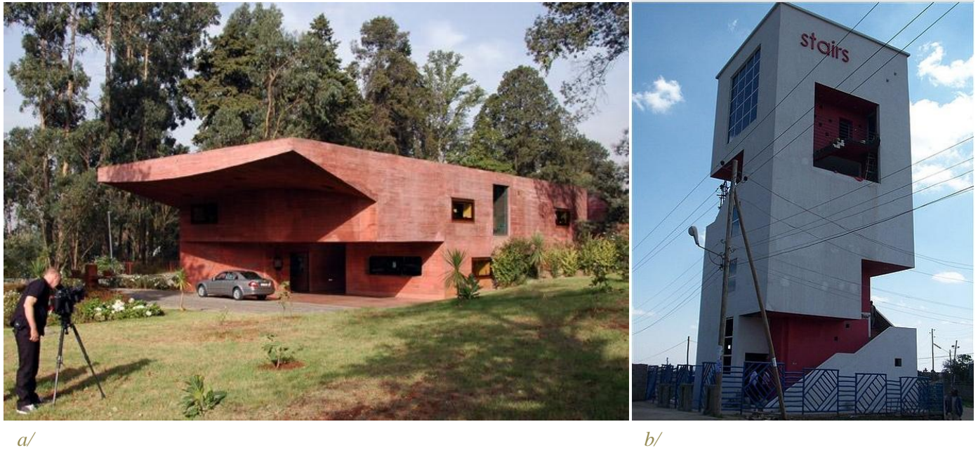
Fig. 4.15 Recent Projects that depict Ethiopian architecture, a) Netherlands embassy b) Stairs Office building
