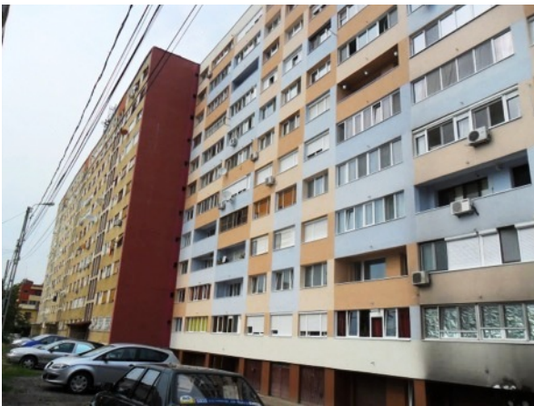
Figure 51 Thermal rehabilitated residential block
