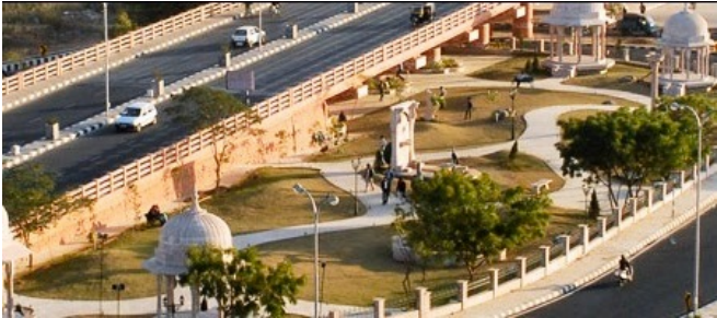
Figure 171 Jaipur Ring Road Development
