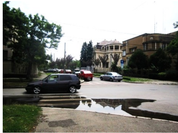
Figure 120 Rain water accumulation on road
