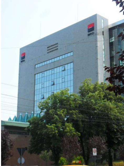
Figure 53 Romanian development bank headquarter
