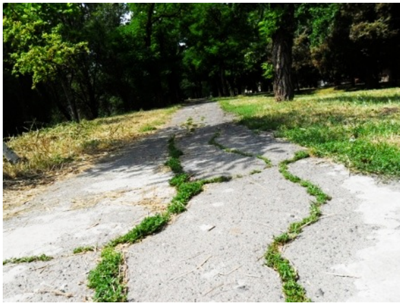
Figure 119 Sidewalk along Bega
