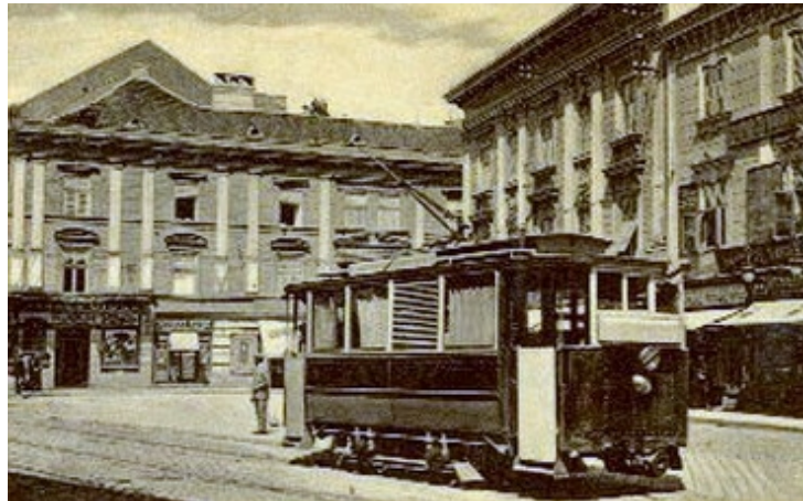
Figure 58 Electric tram around 1899
