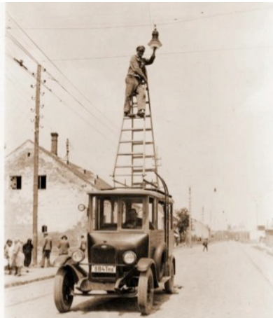
Figure 57 Maintenance electric public light
