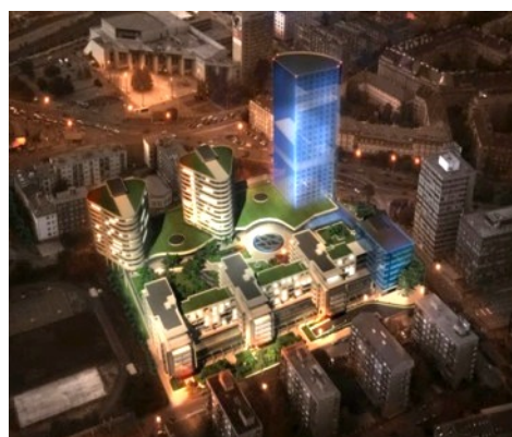
Figure 67 New development in Bratislava
