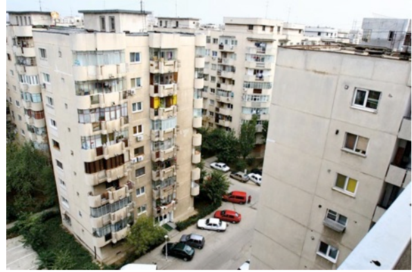
Figure 50 Residential prefabricated neighbourhood
