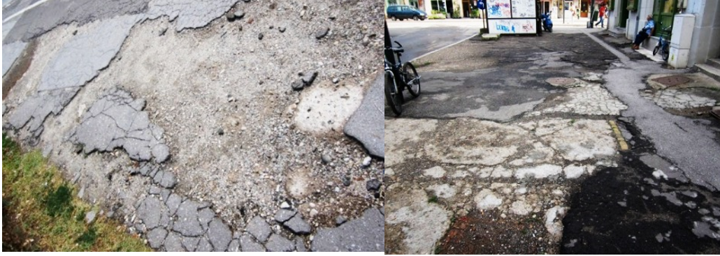
Figure 118 Road & Sidewalk in Fabric
