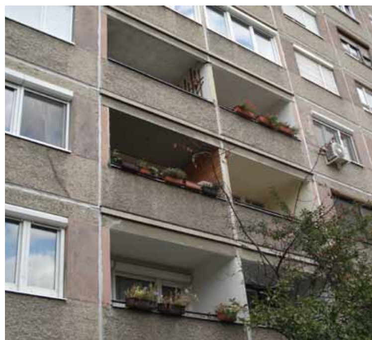
Panel blocks at Kelenföld, XI. district
