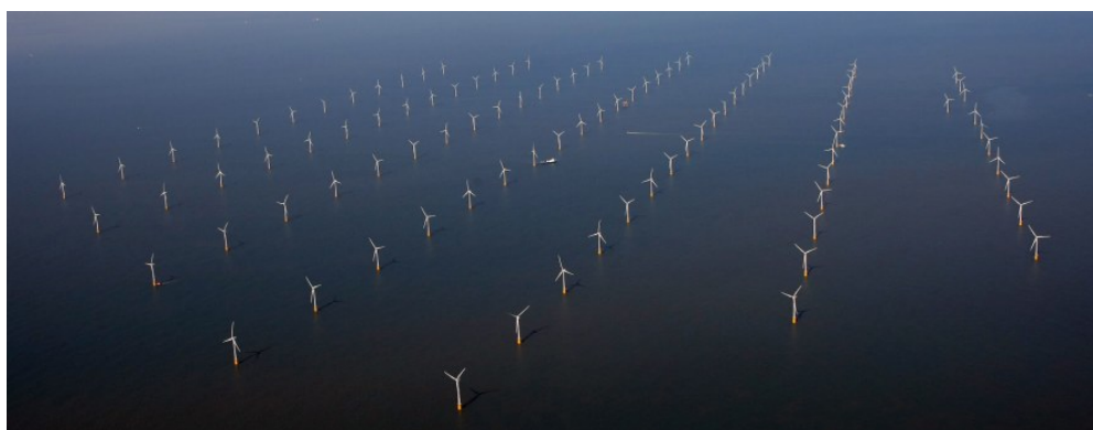
Figura 1.1: Tipica wind farm off-shore
