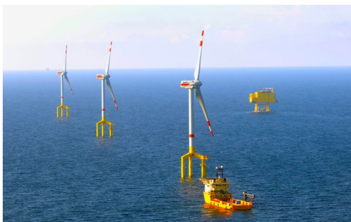
(a) The HVDC Light converter on the BorWin alpha platform with some wind turbines.
