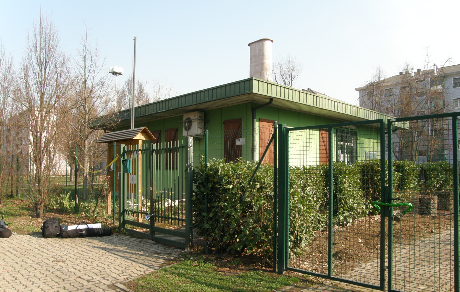
Figure 6.3 External view of La Casetta Verde
