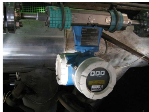
Figure 2.8 Coriolis flow meter.
