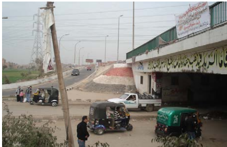
Figure 7.10. Al-Mi'timdiyya ring road exit.
