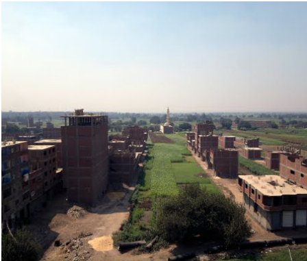
Site Photo- Courtesy of Noheir Elgendy
