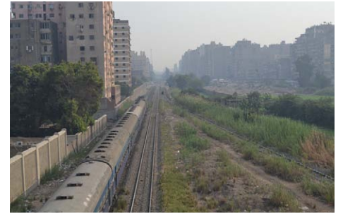
Site Photo- Courtesy of Noheir Elgendy
