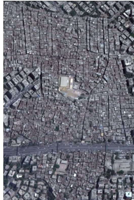
Figure 5.7. Type C: Deteriorated Urban Pockets
