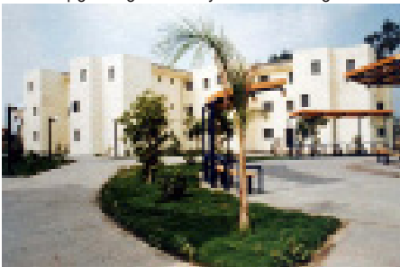
Figure 3.11. Telal Zeinhom project after upgrading. Courtesy of archnet.org
