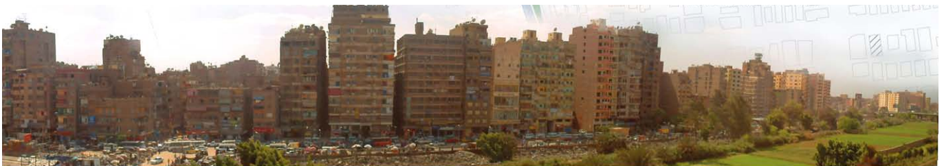
Figure 6.5. Ard al-Liwa Urban Facade
