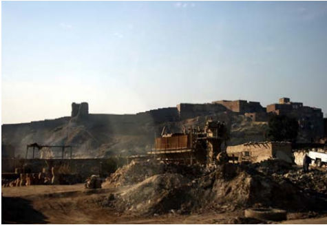
Site Photo- Courtesy of Noheir Elgendy
