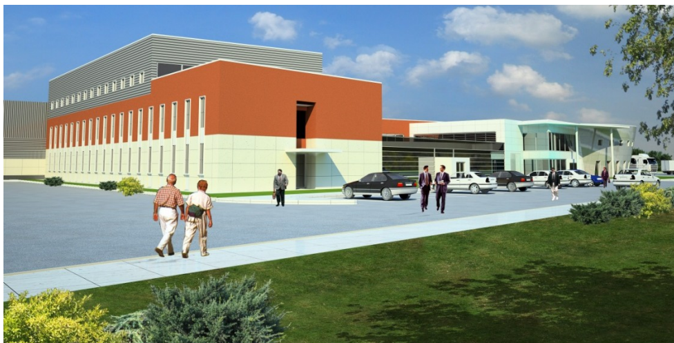
Fig. 6-8: Friterm Factory and office block (First design, before BREEAM, northwest / southwest view)
