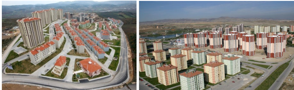
Fig. 5-1: A housing development in Bursa (Left)
