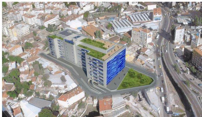
Fig. 6-28: AKPLAZA, Aerial view 60
