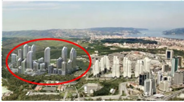
Fig. 5-20: A project development registered to LEED, Maslak 1453, İstanbul 59
