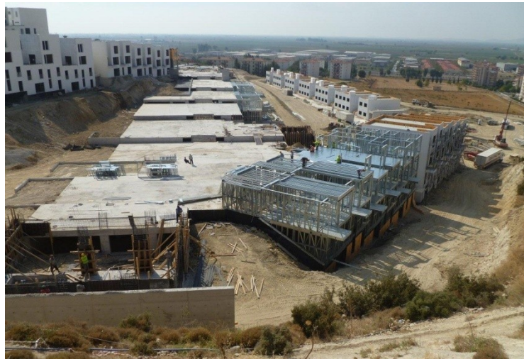
Fig. 6-39: Case study E, Photo from the construction site 76
