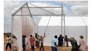
FIG. 3.30: ASSEMBLING OF A WAREHOUSE: RED CROSS TRAINING
