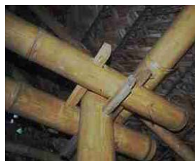
FIG. 6.33: TRADITIONAL BAMBOO JOINT
