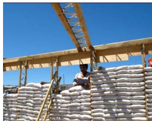
FIG. 6.24: WALLS MADE OUT OF SAND BAGS
