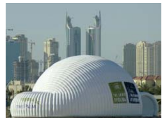
FIG. 5.31: DOUBLE MEMBRANE AIR SUPPORTED PAVILION
