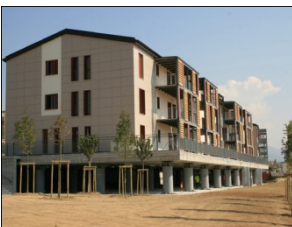
FIG. 6.18: PROGETTO C.A.S.E., NEW NEIGHBOURHOOD BUILT UP AFTER THE EARTHQUAKE
