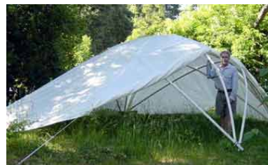
FIG. 6.30: STRUCTURE BASED ON BENT ELEMENTS
