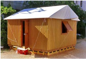
FIG. 6.36: PAPER LOG HOUSE SHIGERU BAN
