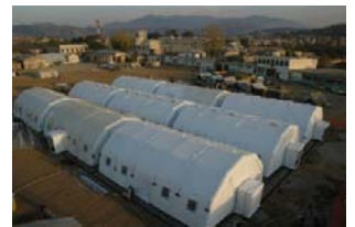
FIG. 4.1: MSF, INFLATABLE HOSPITAL CAMP
