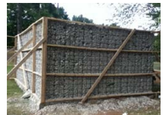
FIG. 6.31: LOAD BEARING WALLS MADE OF RUBBLE
