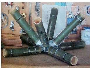
FIG. 6.32: BAMBOO PLUG AND PLAY JOINT
