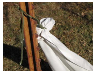
FIG. 6.42: STONE AS REINFORCEMENT FOR TARPAULINS AT CONNECTION POINTS
