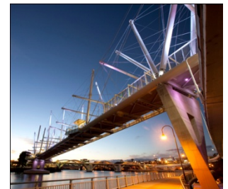
FIG. 3.5: KURILPA PEDESTRIAN BRIDGE, BRISBANE
