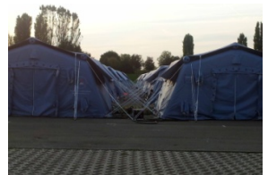
FIG. 2.7: GUY ROPES TO STABILIZE INFLATABLE TENTS
