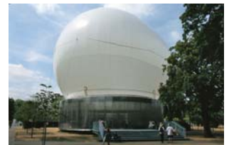
FIG. 7.4: THE FLOATING HELIUM-FILLED ROOF OF THE SERPENTINE GALLERY, OMA 2006
