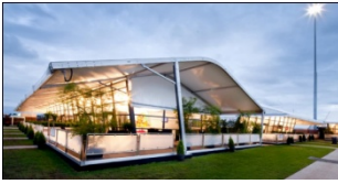
FIG. 4.12: CUSTOM MADE DESIGN MADE WITH MODULAR SYSTEM OF ALUMINIUM FRAME TENTS
