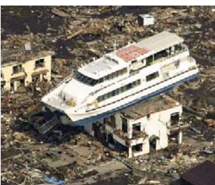
FIG. 0.7: JAPAN TSUNAMI DAMAGES
