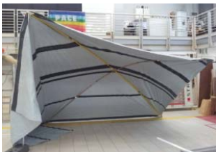
FIG. 3.32: HOW TO INTRODUCE TENSION IN A FLAT TARP, S(P)EEDKITS WORKSHOP 2012
