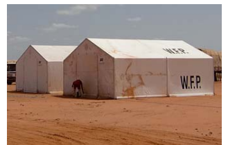
FIG. 5.20: WAREHOUSE WIK HALL"
