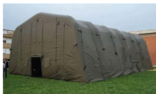
FIG. 5.26: INFLATABLE HANGAR, BY EUROVINIL
