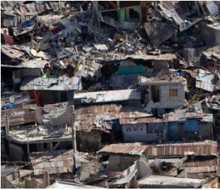
FIG. 0.6: HAITI EARTHQUAKE DAMAGES
