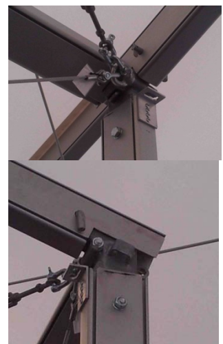
FIG. 4.10-11: ALUMINIUM FRAME TENT, TYPICAL CONNECTIONS
